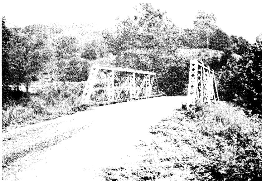
Figure 21. Single-span, low Pratt, half-hip truss bridge in Rockbridge County; built by Variety Iron Works, Cleveland, Ohio; date unknown. (See form/photo number 08-81-15.)
