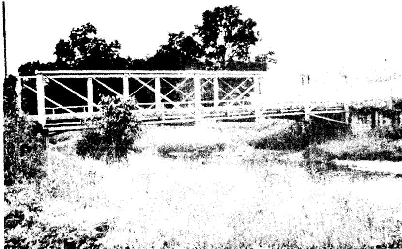
Figure 3. A low Truss Leg bridge with the less satisfactory vertical end posts. (Augusta County; see form/photo number 08-07-14.)
