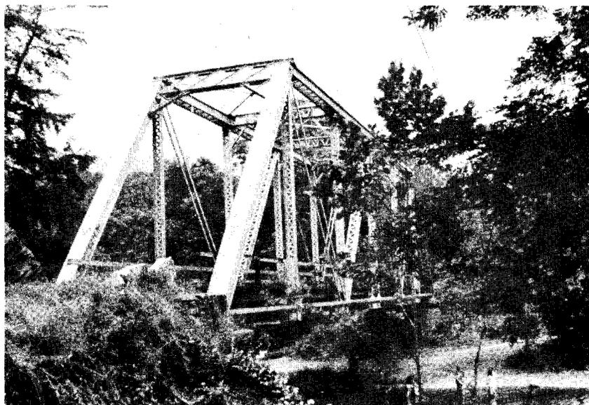
Figure 16. Single span triangular/Warren-type truss in Augusta County with pin connections. Builder and date unknown. (See form/photo number 08-07-30.)
