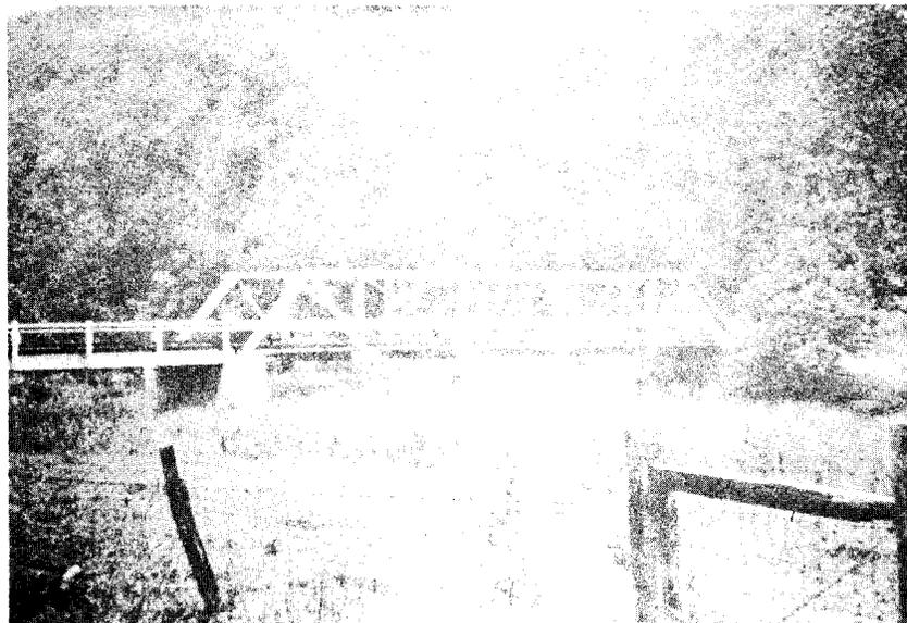
Figure 12. A Low Pratt, half-hip truss whose end posts/batter braces do not bisect a full panel. (Rockingham County; see form/photo number 08-82-18.)
