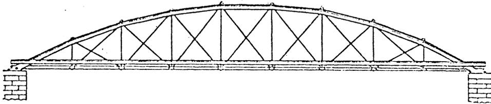
Figures 7 and 8. Squire Whipple's all-iron truss bridges patented in 1847, having cast iron compression members and wrought iron tension members. (From A Span of Bridges, H. J. Hopkins, p. 129.)
