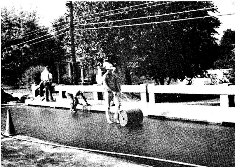
Figure 8. Rolling of the membrane to assure contact with the deck.
