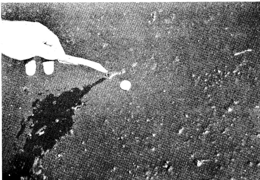
Figure 17. Bubbles in first coat of coal tar epoxy sealcoat.
