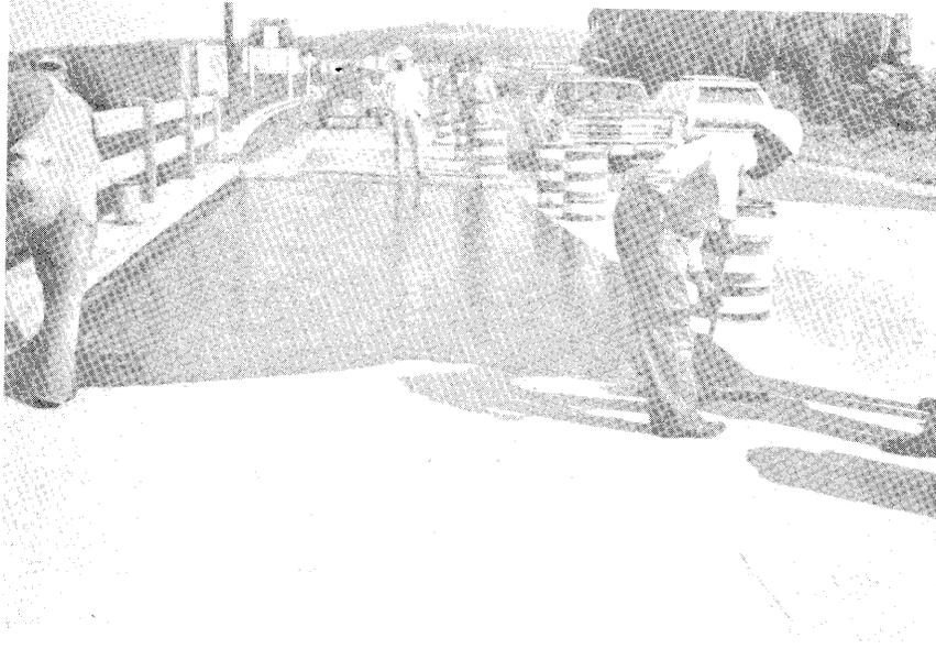
Figure 14. Application of Witmer liquid membrane with squeegees.
