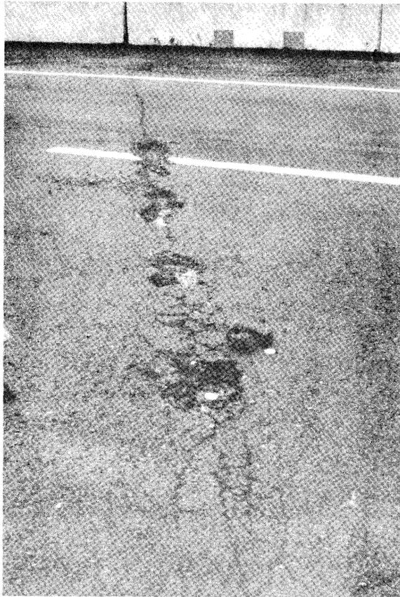
Figure 13. Raveling of asphaltic concrete overlay over deck expansion joints.
