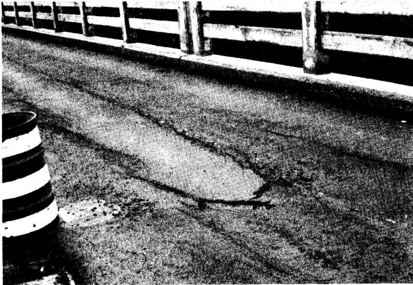
Figure 16. Failure of asphaltic concrete overlay on Witmer membrane.
