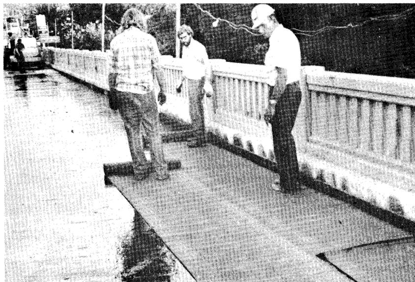
Figure 19. Placement of roofing sheet on Polytok membrane.
