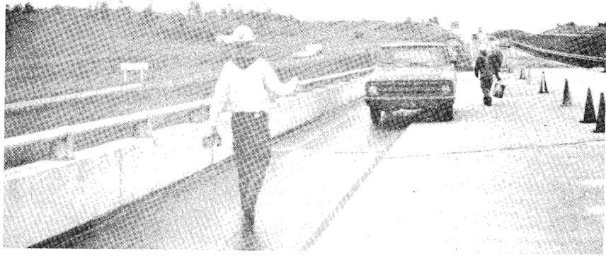
Figure 11. Rolling with light truck to set the laps between adjacent membrane sheets.
