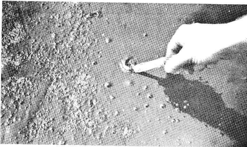
Figure 15. Bubbles in first coat of Witmer membrane.
