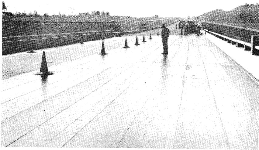
Figure 12. View of completed Protecto-Wrap membrane before paving.
