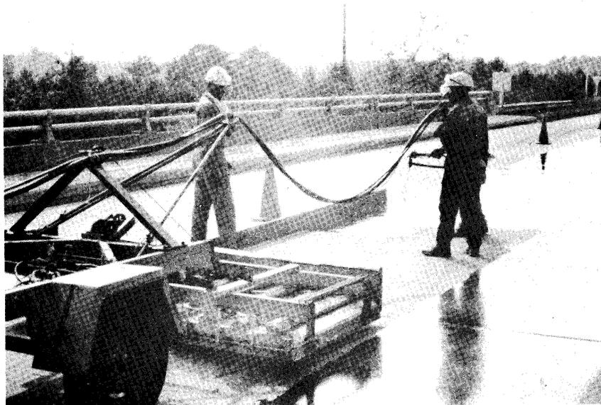
Figure 22. Spray application of Chevron's membrane system.
