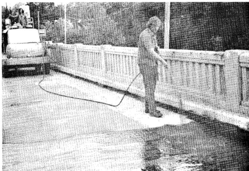
Figure 18. Spray application of Polytok liquid membrane.
