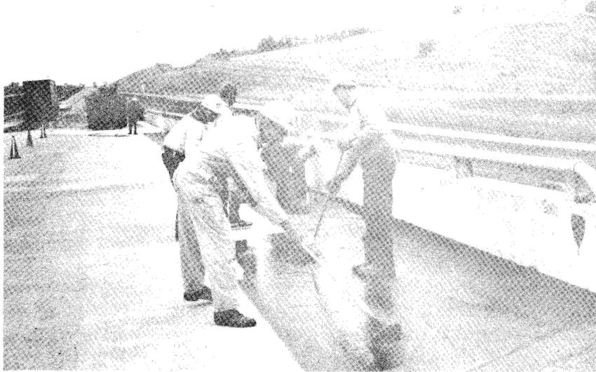
Figure 9. Application of Protecto-Wrap membrane.
