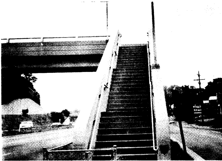
Figure 9. Steps decrease walking distance when compared to ramps but other problems prove them to be less efficient than ramps.
