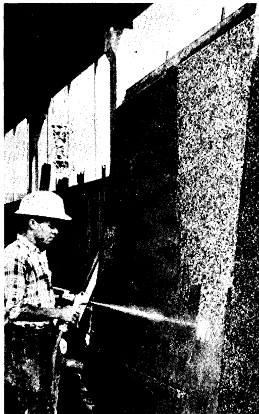
Figure 20. Exposing the aggregate by brushing and washing (Note: This is a precast slab raised from its horizontal casting position and thus washing may begin at any point since the concrete is of the same age and consolidation throughout.)
