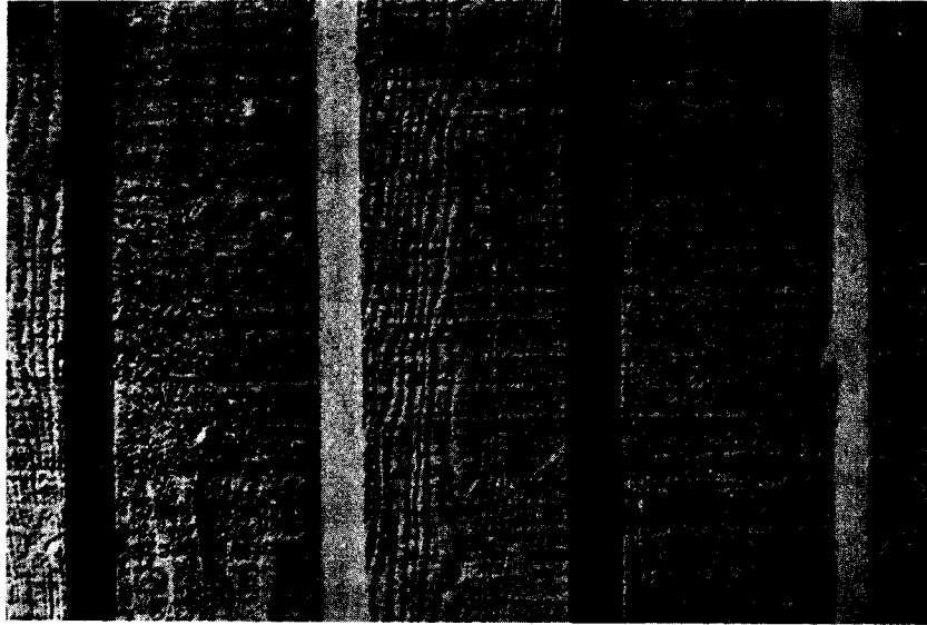
Figure 3. Wood textured finish duplicated from fiberglass forms.
