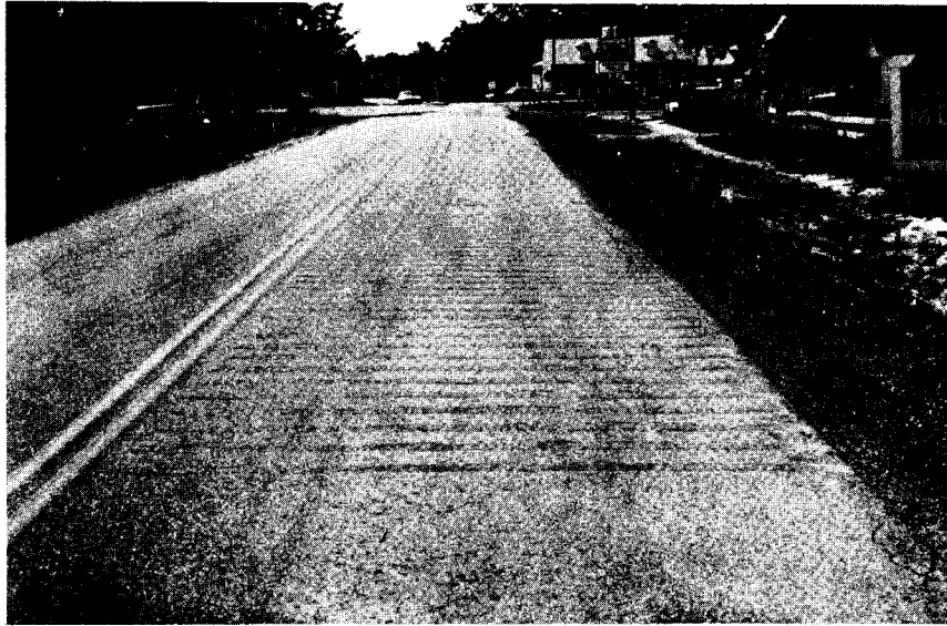
Figure 8. Rumble strips located on Route 606 before the intersection of Route 1.
