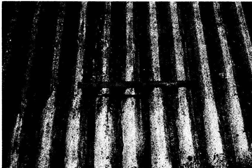
Figure 18. Close view of the rumble strips on gore area.
