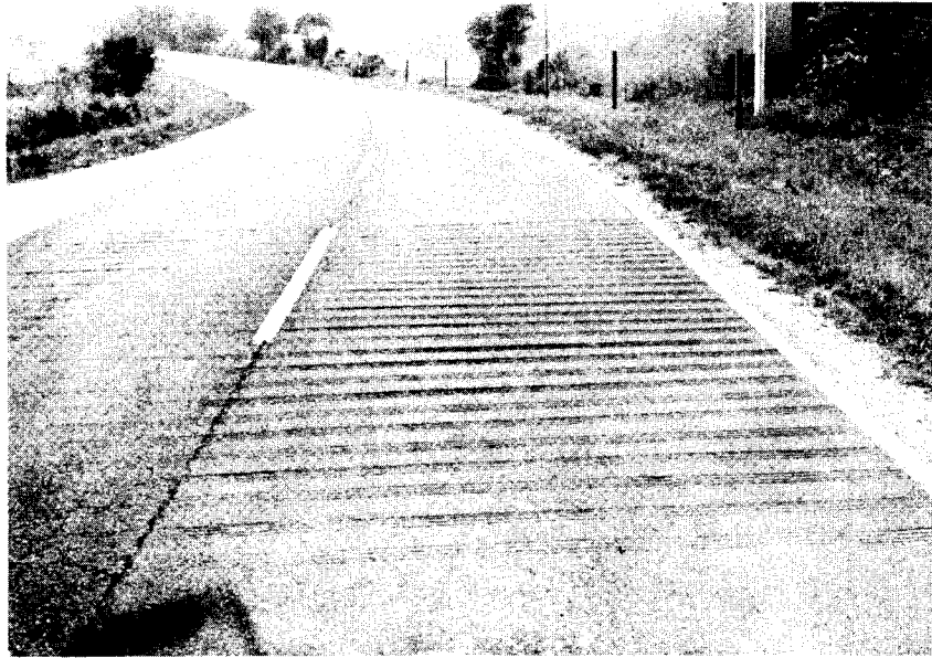
Figure 12. Rumble strips cut into passing lane of Route 29 before Rapidan River. View is opposing traffic direction.
