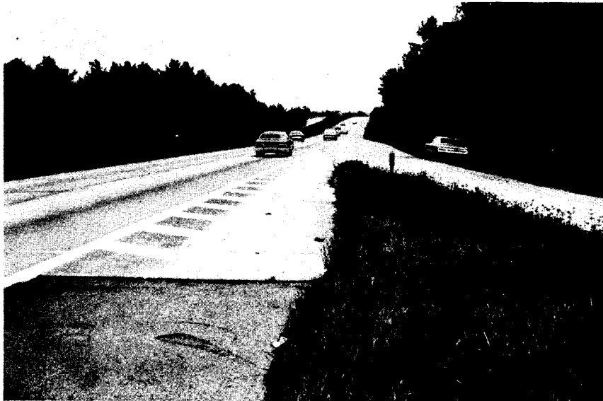
Figure 17. Rumble strips on interstate gore area.
