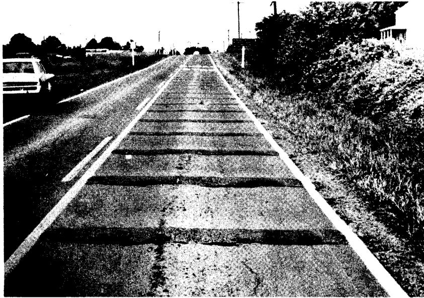
Figure 4. Rumble strips on Route 28 before the intersection of Route 17.
