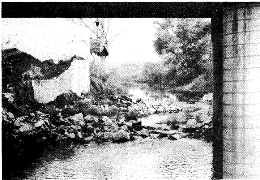
Figure 2. Demolished bridge during cleanup. Note rock berm.
