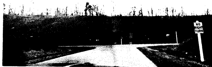
Figure 7(d). Same interchange as in Figure 7(c). View from crossroad. Note the location of the no right turn sign on the extreme edge of the right shoulder.
