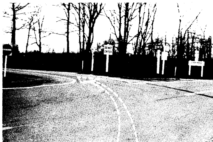
(b) The driver went through the opening in the double yellow lines and entered the wrong way through the right lane of the exit ramp as shown by the arrow. Recommended improvements are: (1) Provision of yellow lines and pavement edge lines as shown in Figure 15; and (2) provision of stop lines.
