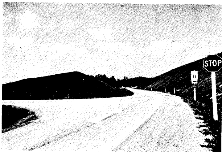
Figure 7(c). View from the exit ramp of the same interchange. The signs have been changed and pavement marking provided. The stop sign and stop line are now on the exit ramp.
