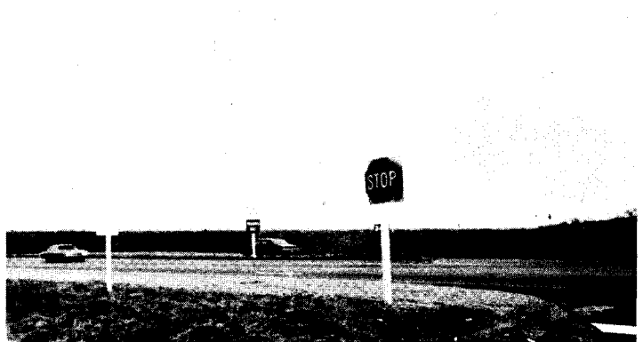
Figure 16(b). Exit ramp of I-95 south and Rte. 1 median. Site of six wrong-way incidents. Left median nose needs to be delineated and median opening reduced as shown in Figure 8(d).
