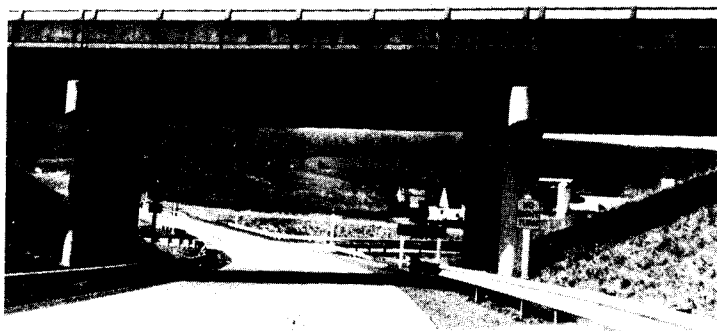
Figure 12(c). Interchange 53A on I-81 — view from crossroad with exit ramp on right across the bridge underpass. Site of two wrong-way entries from crossroad both by drunken drivers. No right turn sign improperly placed. Should be as shown in Figure 12(d). No lane separation marking provided.
