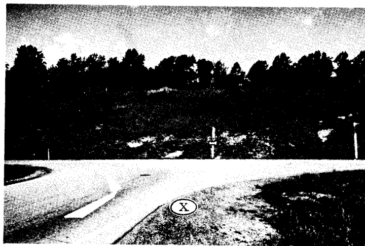
Figure 7(f). The interchange could be further improved by (1) providing left turn arrow on exit ramp in addition to straight arrow as shown on the right, (2) providing left turn arrow on crossroad, (3) placing no right turn sign closer to the pavement edge at x.
