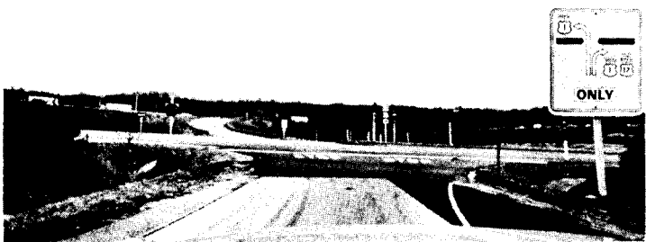
Figure 8(c). Use of intersection geometry sign. Either replace sign in Figure 8(a) by the sign shown above or provide sign in Figure 13(b) on left corner as shown by x in Figure 8(d).
