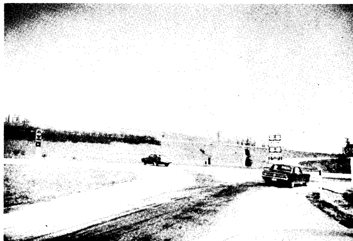
Figure 6(b). Interchange 9 — view from I-81 north exit ramp onto Route 11. Site of wrong-way entry by drunken driver from the crossroad. Channelize left lane by eliminating flare on left and dividing island on right.
