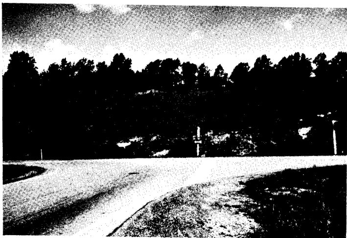
Figure 7(e). View from crossroad closer to the junction with the exit ramp on right and entry ramp on left.
