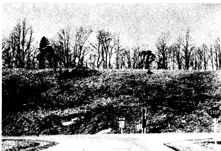
Figure 7(a). Condition after accident — view from crossroad of right exit ramp and left entry ramp. Note stop sign on crossroad and low height of no right turn sign.
