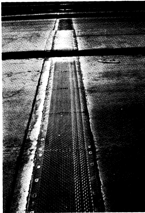
Figure 1. View of an old model Transflex 400 joint with the "honeycomb" type surface texture. (Rte. 154 over Jackson River.)
