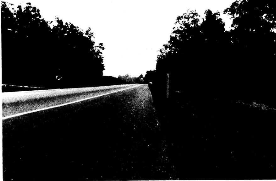
**Figure 1.** Untreated shoulder, southbound direction, Interstate 95.
