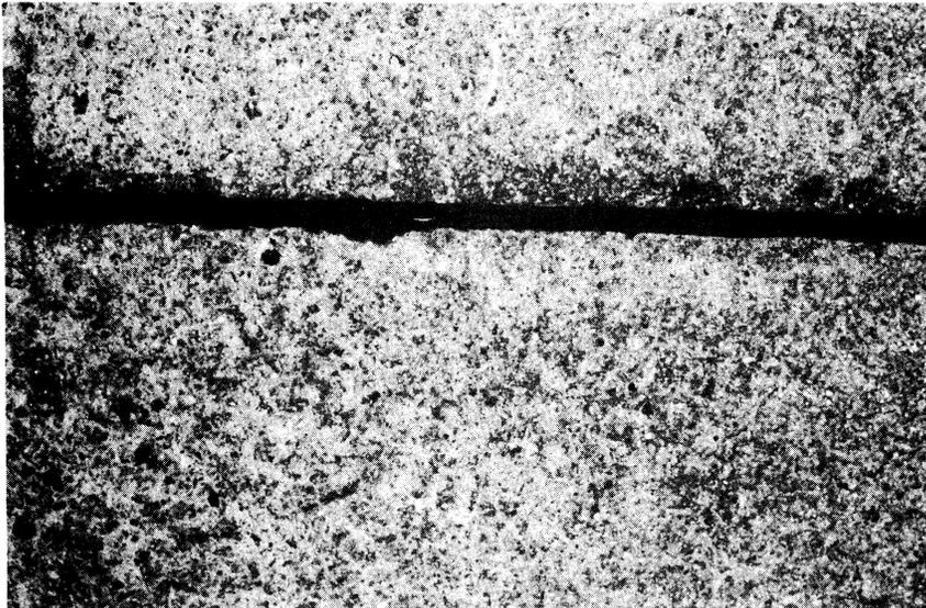
**Figure 6.** Examples of good (upper picture) and poor performance of polysulfide joint sealants on I-95, Emporia.
