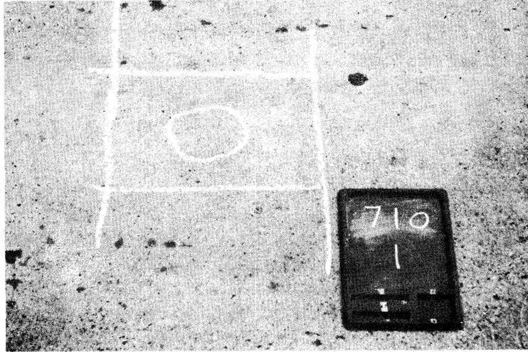
Figure 10. Core location on northern project showing healthy looking pavement, apparently free of scaling and cracks.
