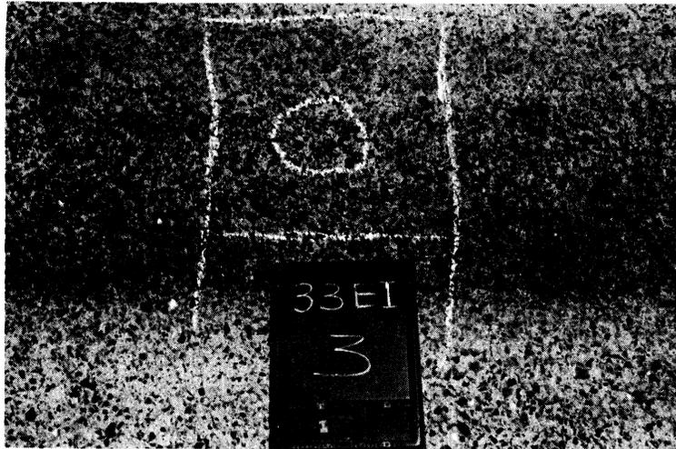
Figure 2. Typical view of severely scaled area in northern project.
