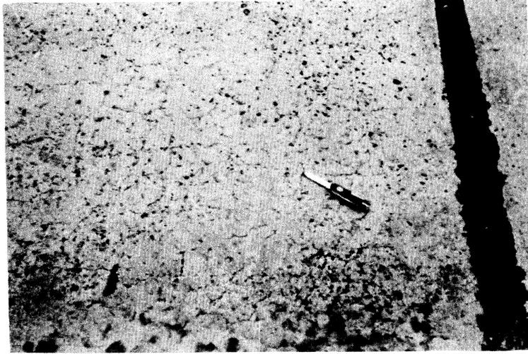
Figure 3. Typical view of pattern cracking on northern project.
