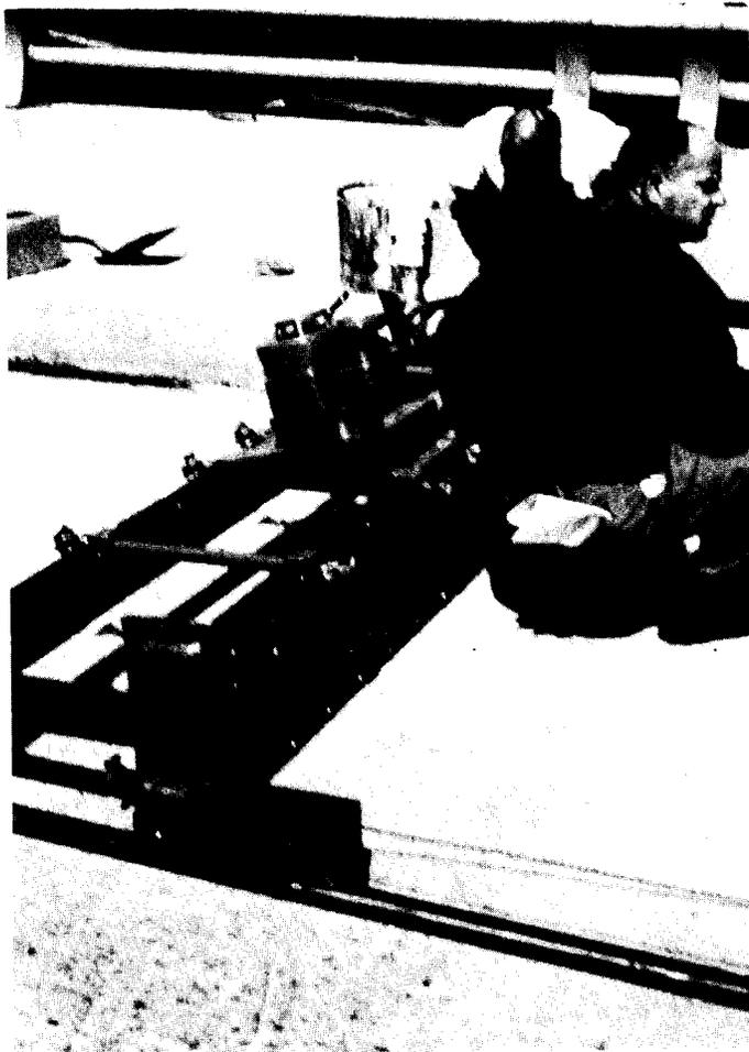
Figure 10. Screed used to finish the top surface of the Guardkote 250 mortar overlay.
