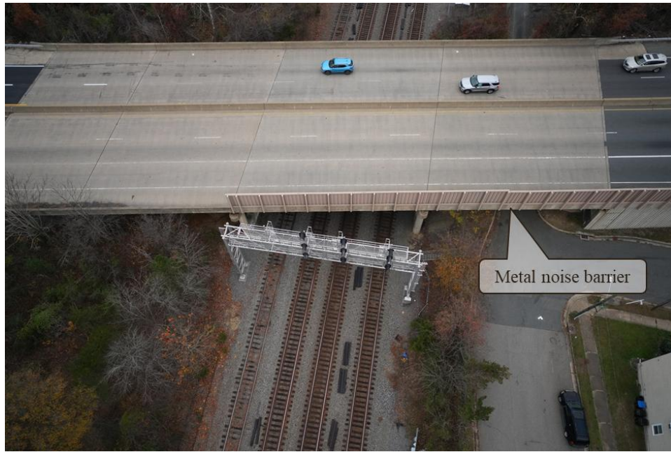
Figure 23. Oblique Imagery from the Fredericksburg Site Showing Metal Noise Barrier, Railroad Tracks, and Truss Structure over Railroad Tracks
