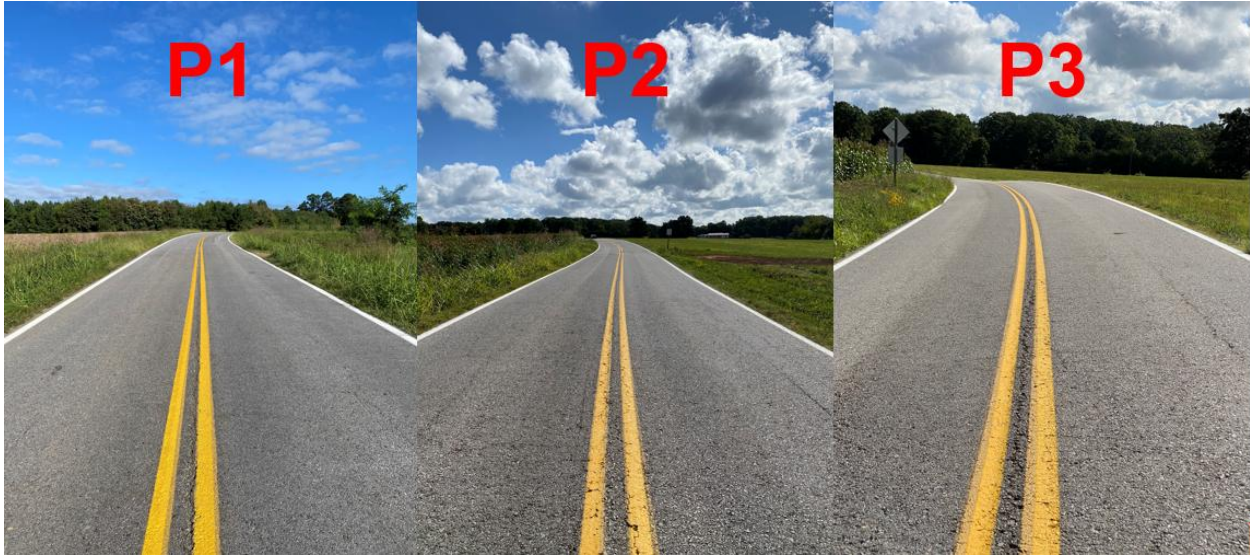
Figure 23. Images of Surface Appearance Approximately 12 Months after Spray-on Rejuvenator Application for Route 750. P1–P3 denote segments receiving spray-on rejuvenator application.
