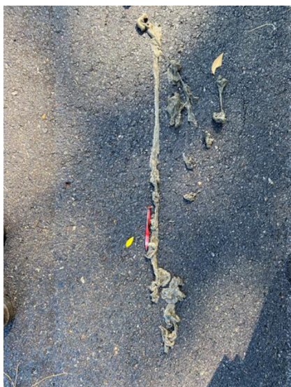
Figure 9. Formation of Polymer Balls on the Pavement Surface Following Premature Vehicle Entry and Braking within the Treated Lane during the Curing Period
