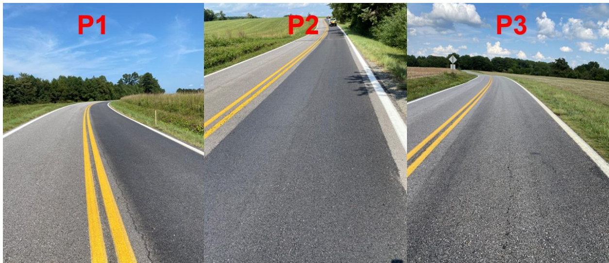
Figure 11. Images of Surface Appearance Shortly after Spray-on Rejuvenator Application for Route 750. P1–P3 denote segments receiving spray-on rejuvenator application.
