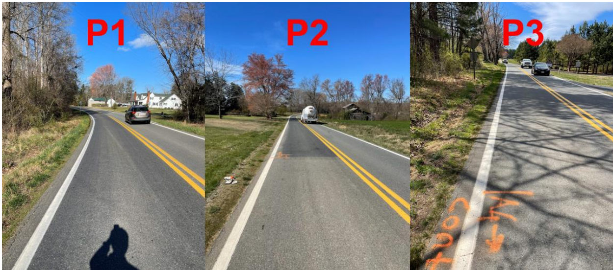
Figure 20. Images of Surface Appearance Approximately 6 Months after Spray-on Rejuvenator Application for Route 640. Treated lane is shown on the left, and untreated lane is shown on the right. P1–P3 denote segments receiving spray-on rejuvenator application.
