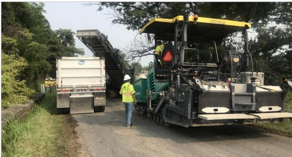
Figure 6. Paver-Laid Full-Depth Reclamation Project on Pitzer Road in Roanoke County
