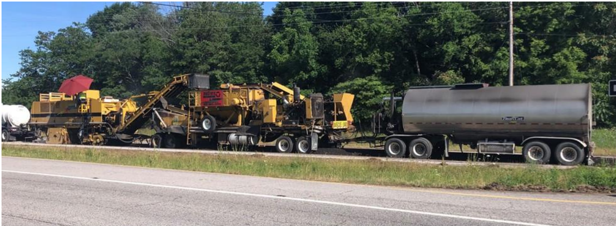
Figure 8. Multi-Unit Cold In-Place Recycling Train
