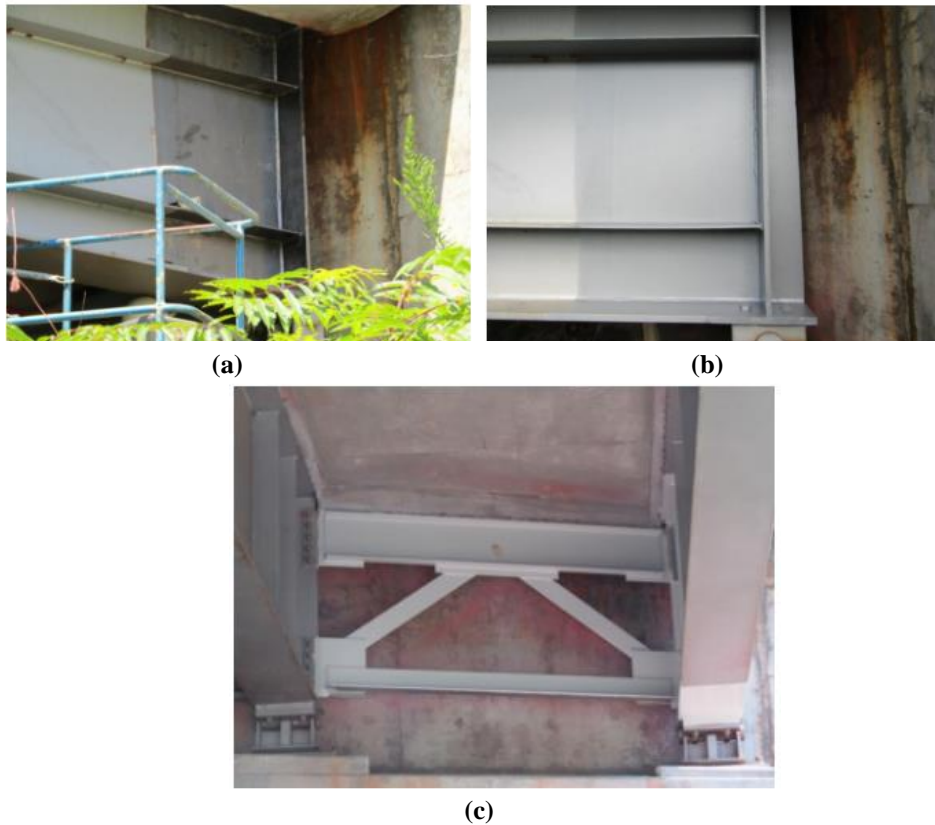
Figure 17. Laser Ablation Coating Removal and Recoating of Route 695 Bridge in August 2017 Showing: (a) After Coating Is Removed on Facia Girder Using Laser Ablation Coating Removal; (b) After Prime Coat Is Applied to Facia Girder No. 4 at Abutment B; (c) After Finish Coat Is Applied to Cross Frame between Girders No. 3 and 4 and to the Bottom of Girder No. 4.
