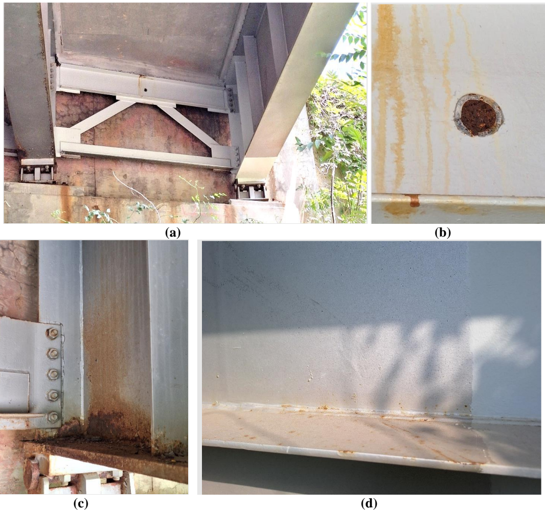
Figure 18. Examples of Areas Cleaned with LACR Alone and Recoated and Areas that Were Not. (a) The girder on the left (girder no. 3, near abutment B) was not cleaned and recoated, whereas the cross frame and girder end on the right (girder no. 4, near abutment B) were cleaned with LACR and recoated. (b) Magnified view of stain and uncoated test area on recoated steel cross frame is also seen near the top of the cross frame, shown in (a). The stain is due to a leaking joint, allowing moisture to seep between the bottom of the end bolster and the top of the secondary member interface because of the failed joint. The uncoated corroded area in the middle of the photo was intentionally left uncoated as part of the first study to observe a LACR cleaned but uncoated area over time. (c) Coating loss and exposed steel are shown where LACR repair would benefit the bridge by mitigating steel loss on the bottom flange and web at the bay 2 side of girder no. 3 near abutment B. (d) The transition on exterior girder no. 4 near abutment B from the original coating to the LACR cleaned and recoated area illustrating how the old coating has numerous small rust sites. LACR = laser ablation coating removal.
