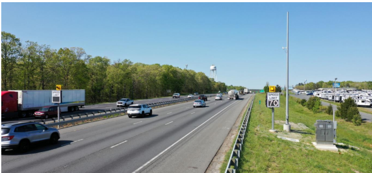
Figure 2. Example of Variable Speed Limit Installations Along the Corridor
