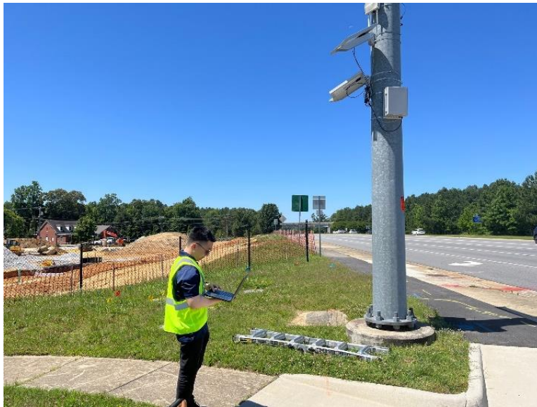
Figure 45. Manual On-Site Intervention to Resolve Gateway #2 Connectivity Issues
