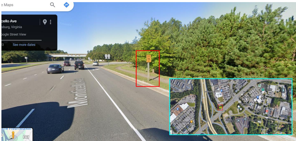
Figure A6. People Counter Installation Location #6: 37°16'27.4"N 76°45'03.7"W, Monticello Ave Westbound
