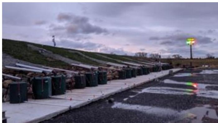
**Figure 40. Completion of the connection of the collection tanks to the collection pipes, which are connected to the edg drains at each section**
