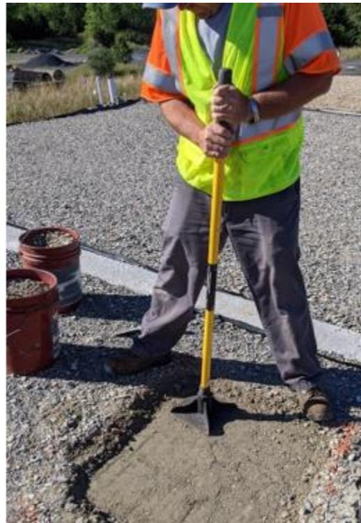
**Figure 11. Compacting the base course material back onto the edg drain geotextile**
