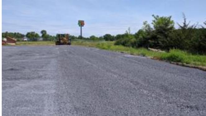
**Figure 27. Placement of crusher run as subbase**
