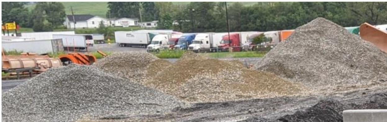
**Figure 55. A photo of the stockpiled base course materials on site during construction**
