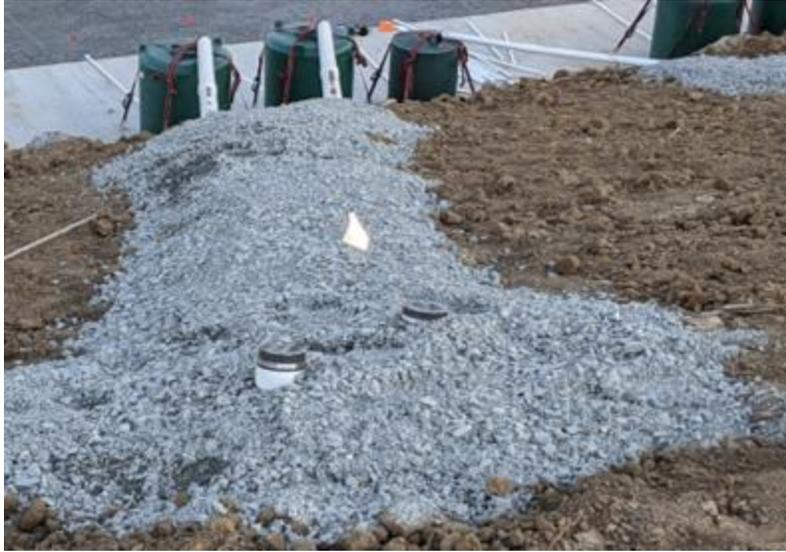
**Figure 35. Completion of the borescope T connectors along the slope and connection of the collection pipes and tanks at each section, located downslope from the test site**
