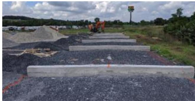
**Figure 28. Construction of curb wall dividers**
