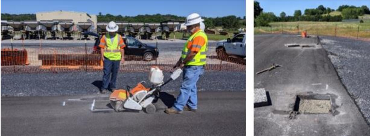
**Figure 8. Marking the pavement and cutting the asphalt overlay to exhume geotextile samples from paved sections**
