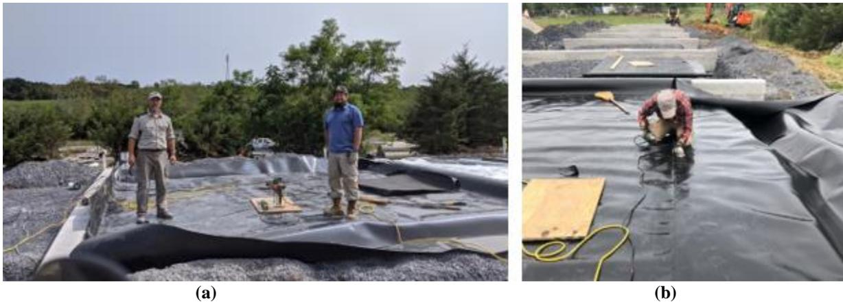
**Figure 31. Installation of the geomembrane hydraulic barrier (a) covering the entire section, and (b) the pieces are being welded together**
