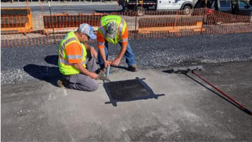
**Figure 12. Placing the asphalt block back onto the recompacted base course aggregate**
