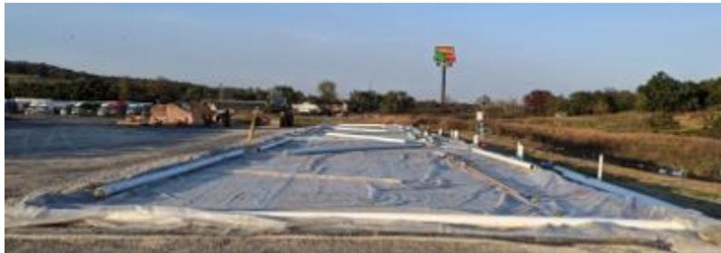
**Figure 36. Plastic sheets being placed over the entire site until the placement of the asphalt overlay**
