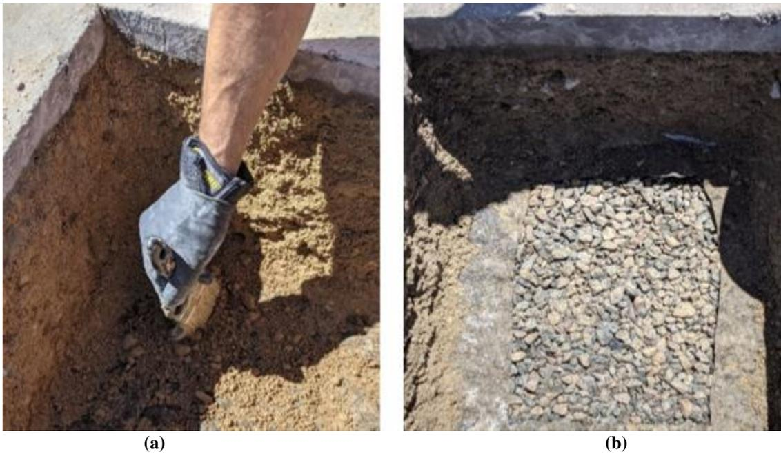
**Figure 9. Removing the base course material and (a) brushing the surface of the geotextile and (b) cutting a sample piece from the exposed geotextile**
