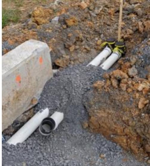
**Figure 30. Installation of collection pipes at the end of the edg drain trenches prior to the installation of the geomembrane liner**
