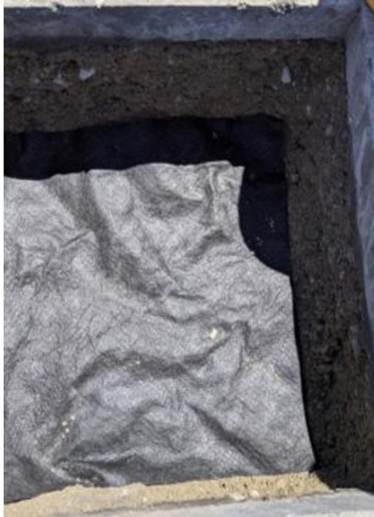
**Figure 10. Placing a piece of new geotextile over the cut area before placing the base course material back onto the edg drain geotextile**
