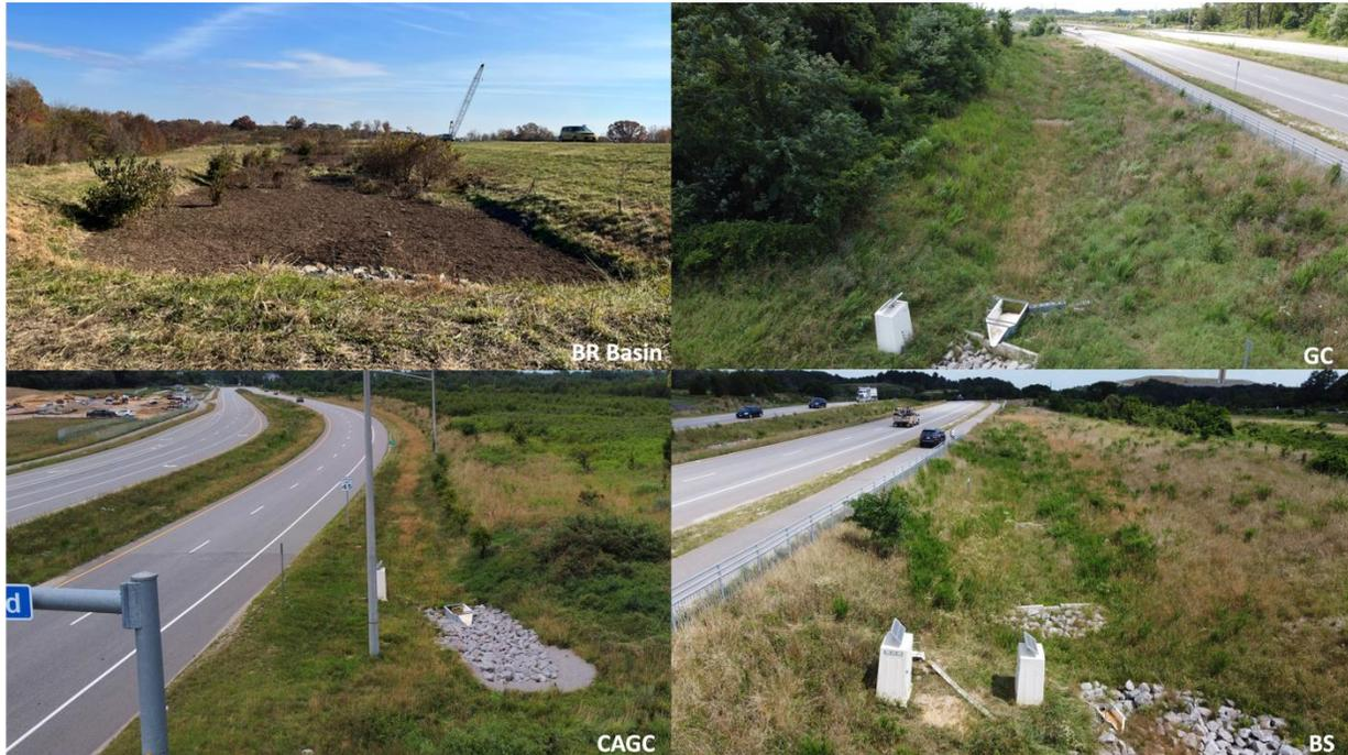
**Figure 4. Four monitored LID designs along Lorton Road (BR: bioretention; CAGC: compost-amended grass channel; GC: grass channel and BS: bioswale)**
