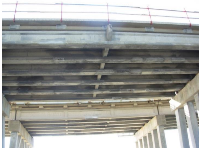
Figure 1. Typical Deterioration on the Lesner Bridge
