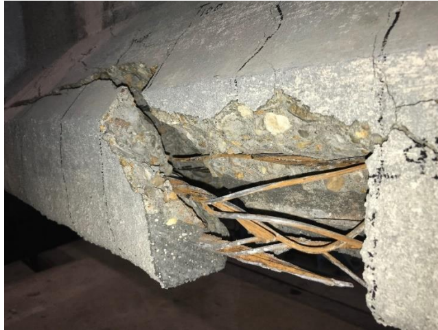
Figure 57. Corrosion-Damaged Strands in and above Patch in I-Beam 3
