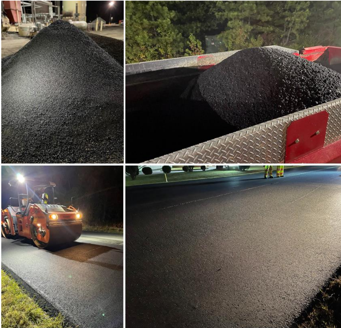
Figure 4. Photographs Taken for Production Operations at the Plant and Paving/Construction in the Field for RPM and Reference Mixtures
