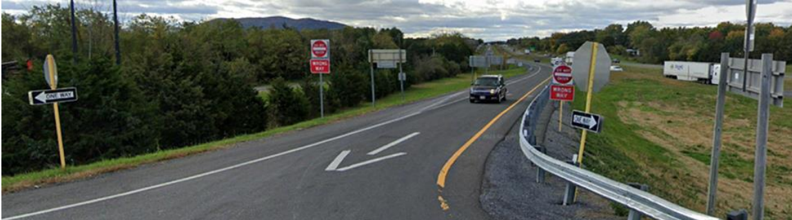
Figure 32. DO NOT ENTER and WRONG WAY Signs, Dual Mounted ONE WAY Signs, and Wrong Way Arrow (Google Street View)
