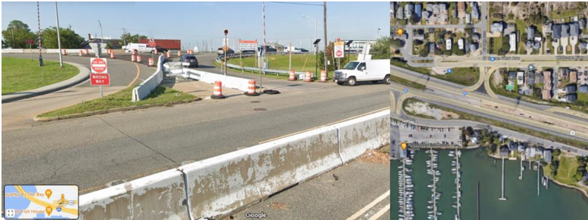
Figure 15. I-64 West Exit 272 Ramps (Google Street View, July 2023)
