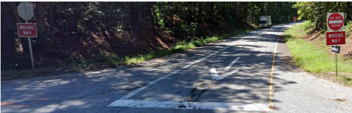
Figure 33. DO NOT ENTER and WRONG WAY Signs, ONE WAY Sign, Stop Bar and Wrong Way Arrow (Google Street View)
