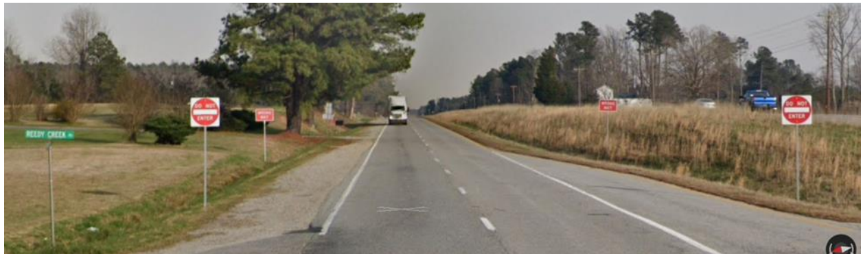
Figure 28. Route 58 Westbound at the Reedy Creek Road Intersection Showing Dual Mounted DO NOT ENTER and WRONG WAY Signs (Google Street View, March 2023)
