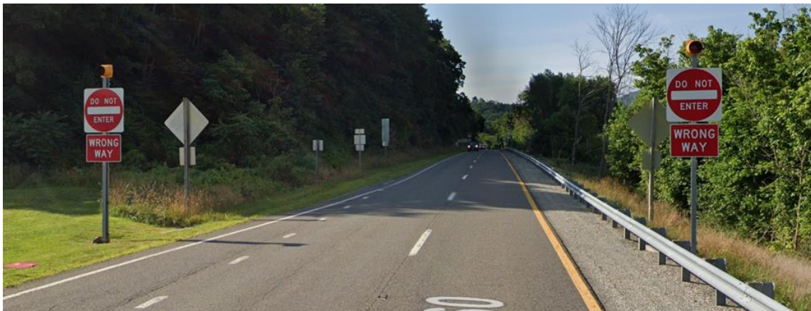
Figure 34. Wrong-Way Driving Detection System on Route 460 at Rich Creek in Salem District (Google Street View)
