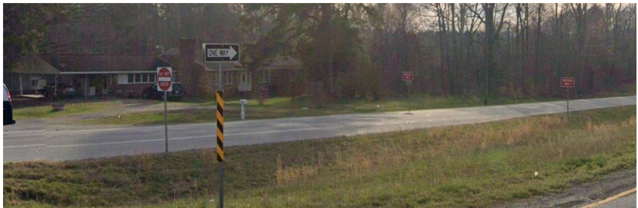
Figure 29. Route 58 Eastbound at the Reedy Creek Road Intersection Showing DO NOT ENTER and Dual Mounted WRONG WAY Signs (Google Street View, March 2023)
