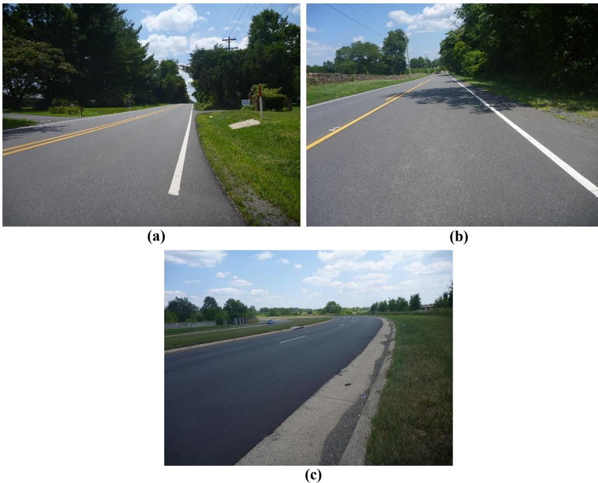
**Figure 53. Photographs of Mixtures: (a) Section 19-A-V, 4 years post-paving; (b) Section 20-A-2, 3 years post-paving; (c) Section 22-A, 1-year post-paving.**
