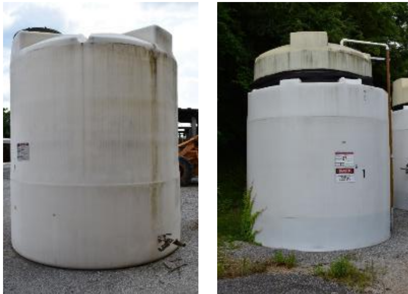
Figure 1. Examples of single-walled (left) and double-walled (right) high-density polyethylene above ground storage tanks managed by VDOT
