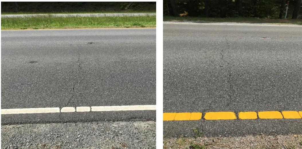
**Figure 10. Reflective Cracking Observed on US 60 After 2 Years**
