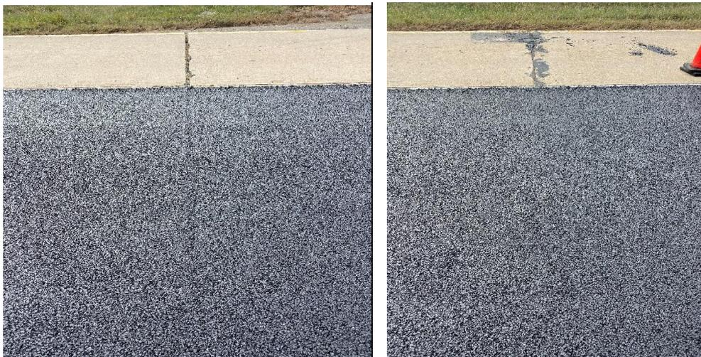
**Figure 11. THMACO Layer Showing Shadow of Concrete Pavement Joint. THMACO = thin hot mix asphalt concrete overlay.**
