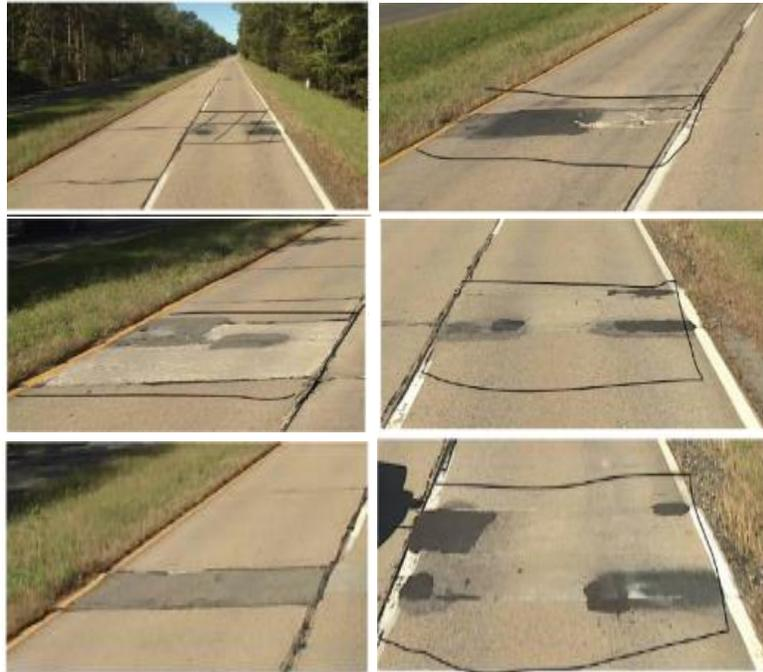
**Figure 2. Existing Pavement Distress on US 60 (New Kent County)**
