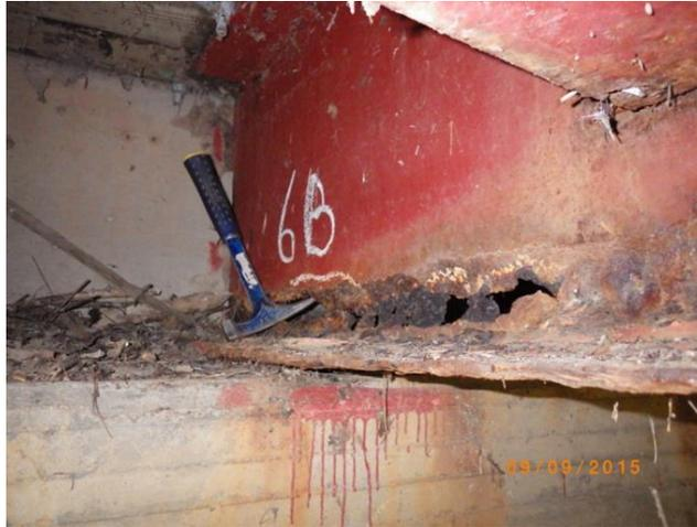
**Figure 1. Example of Extensive Beam End Corrosion Damage**
