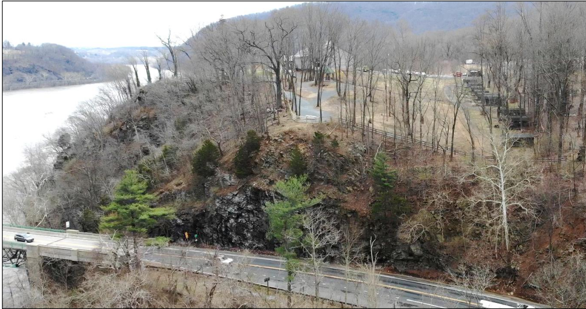
Figure 5. UAS photograph of the east end of Site #4, Route 340 at Harpers Ferry. Center left shows a pod of competent rock where stability is controlled by joint sets. The rock mass changes to softer weathered rock and soil moving to the right (west) causing stability to be controlled by the strength of soil and soft rock.
