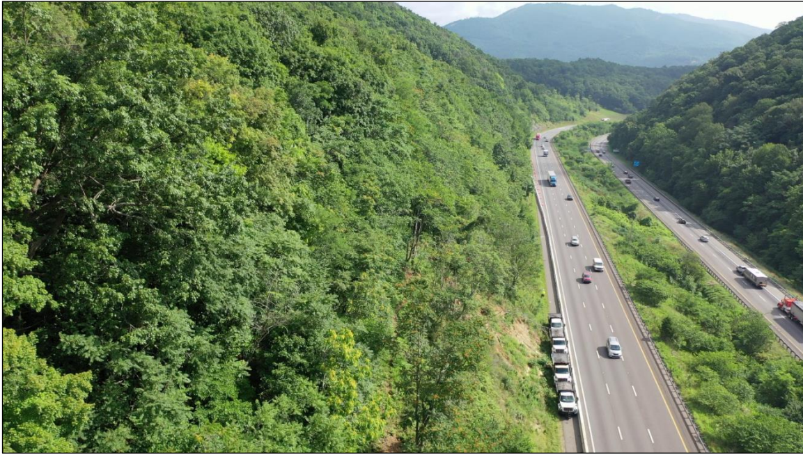
Figure 7. UAS photograph of Site #6, I-81 at MP 126.5 southbound, looking northbound. The current landslide is adjacent to the trucks placed as temporary rockfall barriers. The site of a massive 1969-70 landslide is at, and rising to the left above, the grassy area just beyond the curve in the distance at about MP 127.0. This picture illustrates the challenging nature of the site for UAS flights: dense leaf-on vegetation, narrow valley, rugged median sloping down toward the northbound lanes.
