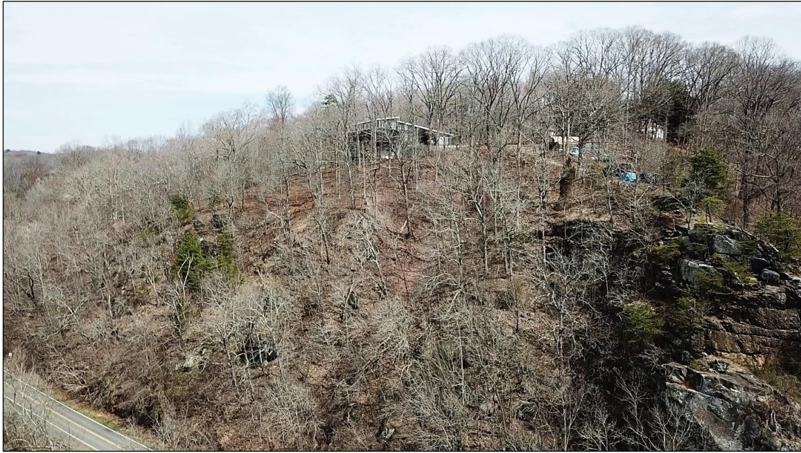
Figure 4. UAS photograph of Site #3, Route 685 River Road Lynchburg. Right side shows large rocky slope face with potential block failures controlled by the structural geology.
