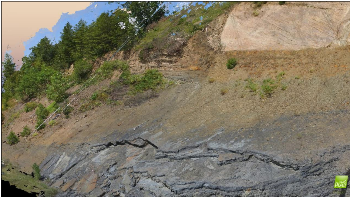
Figure 24. Site #2, Deerfield. UAS point cloud, scaled and georeferenced for obtaining measurements including the extraction of geologic structure data for stability analyses. This model represents conditions in 2016, prior to rock block failures from the rock projection feature in the top center of the image. This is a portion of one of the two point clouds used to test change detection techniques to fulfill of Task #11.
