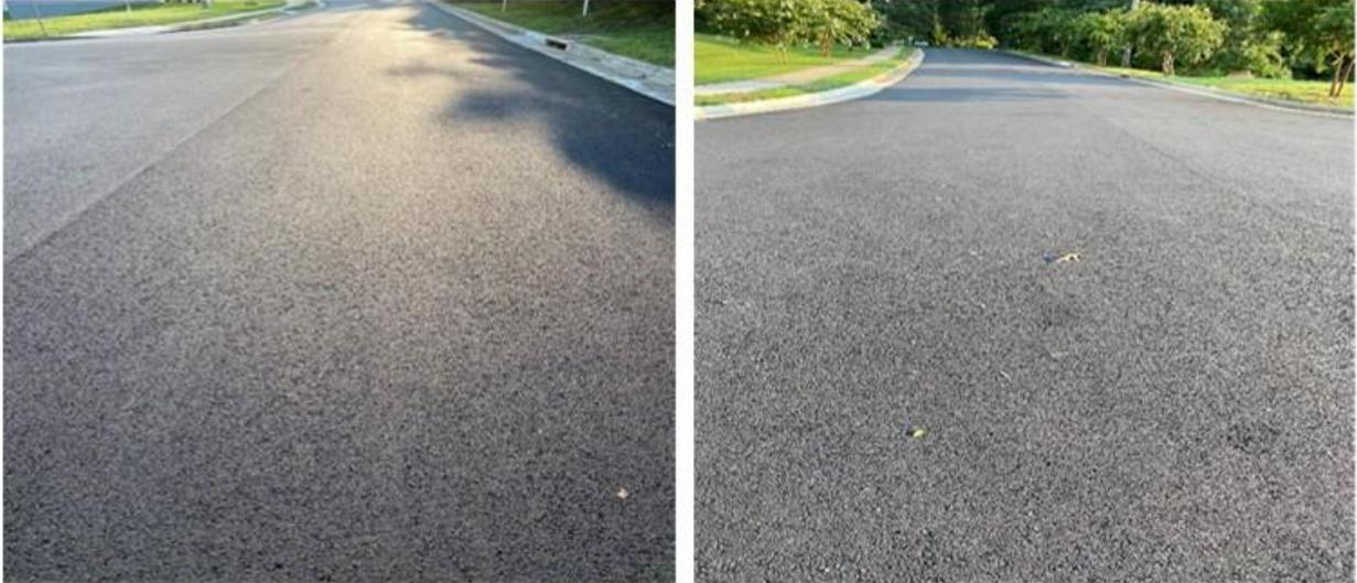
**Figure 12. FDR + 2-in AC Surface at Estates at Leeland, Spotsylvania County, 1 Year After Construction. FDR = full depth reclamation; AC = asphalt concrete.**
