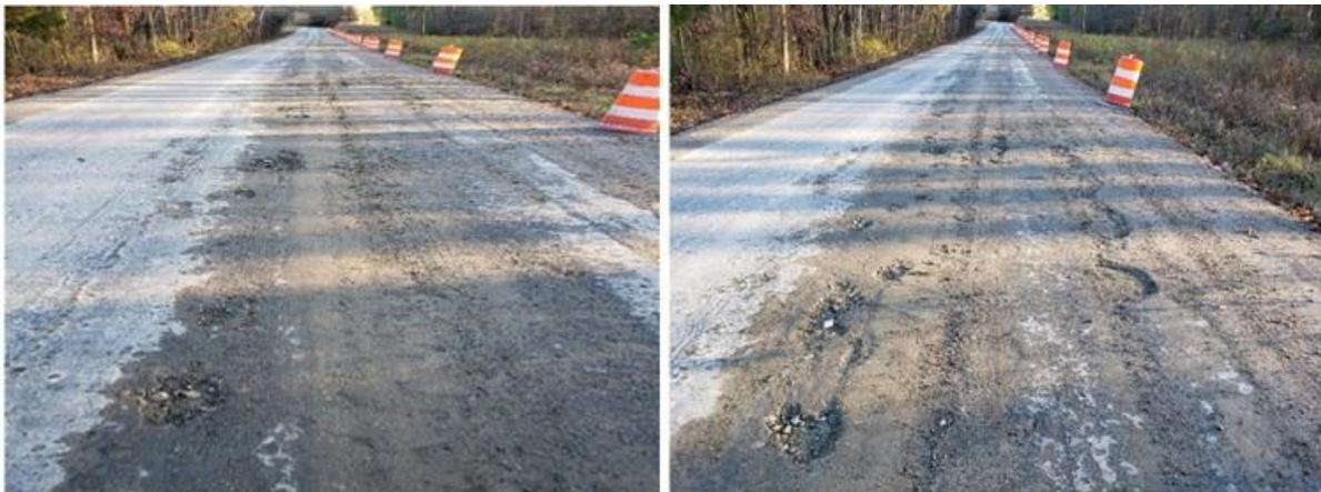
**Figure 3. First FDR Trial Section on Rte. 602. FDR = full depth reclamation.**
