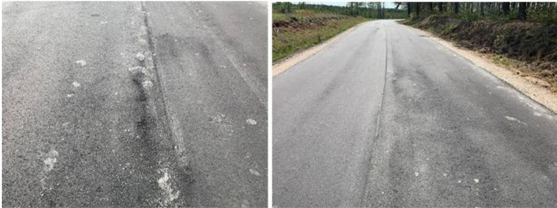
**Figure 4. Segregation and Raveling on SM-9.0 Mix Placed Over Second FDR Trial. FDR = full depth reclamation.**
