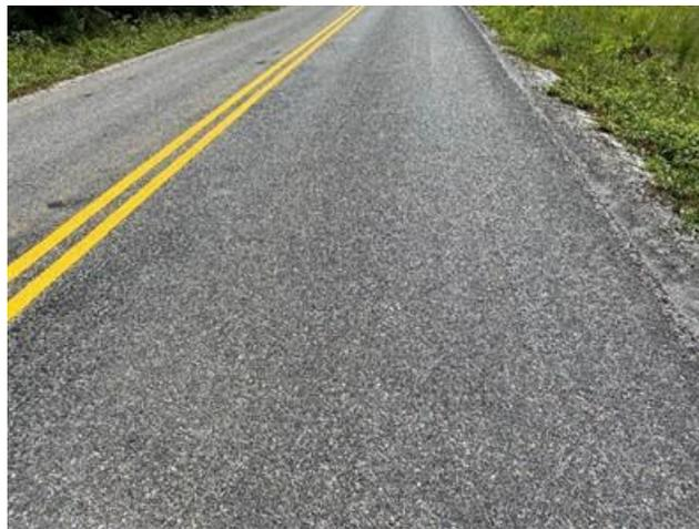
**Figure 10. FDR + Blotted Seal Coat, 1.5 Years After Construction. FDR = full depth reclamation.**
