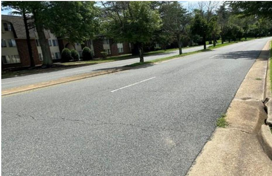
**Figure 14. FDR + 2.5-in AC Surface on Stonewall Parkway, 8 Years After Construction. FDR = full depth reclamation; AC = asphalt concrete.**
