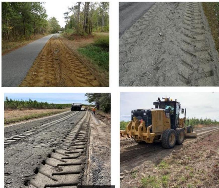
**Figure 5. FDR Process on Rte. 602. FDR = full depth reclamation.**
