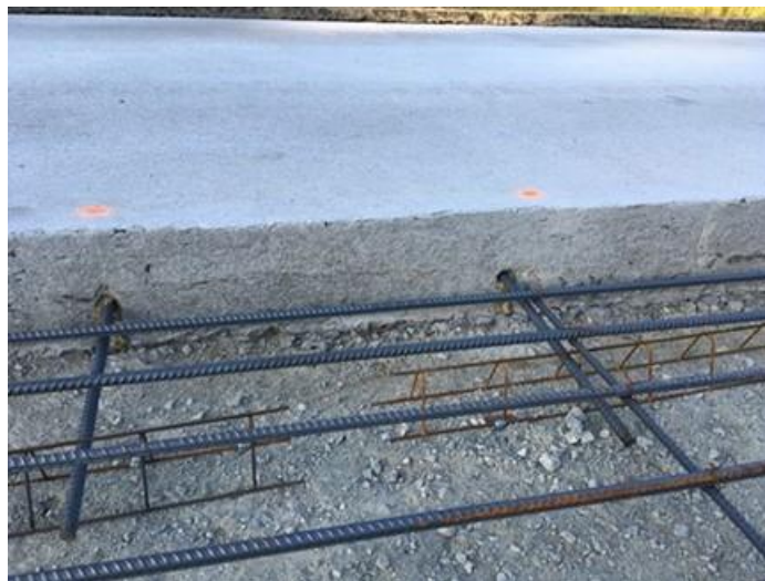
Figure 11. Drilled and Epoxied Tie Bars to Right Lane
