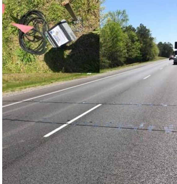
Figure 18. Traffic Data Collection Tubes on US 60W
