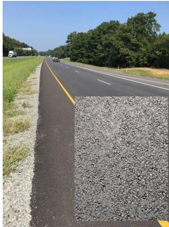
Figure 20. Composite Pavement SMA Surface Condition After 2 Years of Traffic. SMA = stone matrix asphalt.
