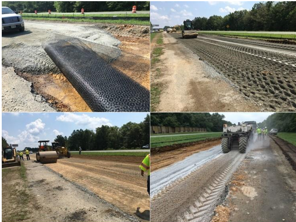
Figure 6. Base Removal, Replacement, and Stabilization
