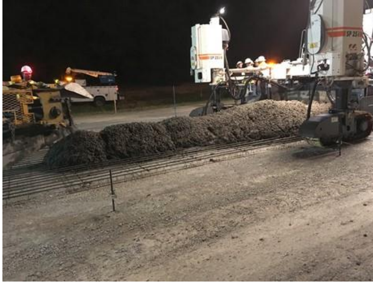
Figure 8. Paving Right Lane With a Slipform Paver
