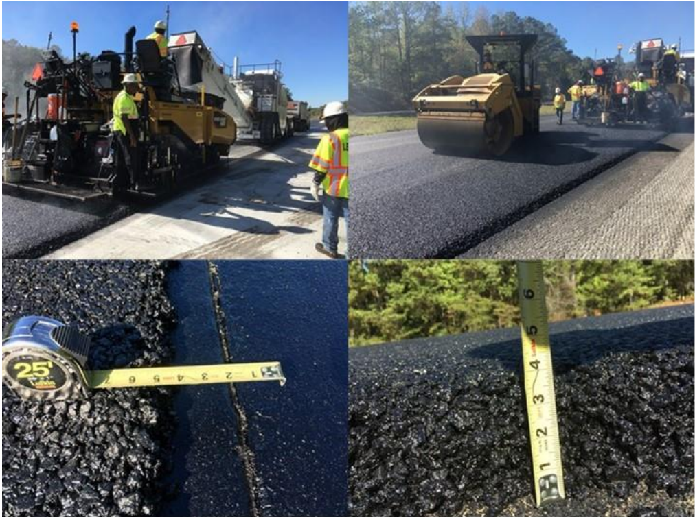
Figure 13. SMA Overlay Operation. SMA= stone matrix asphalt.
