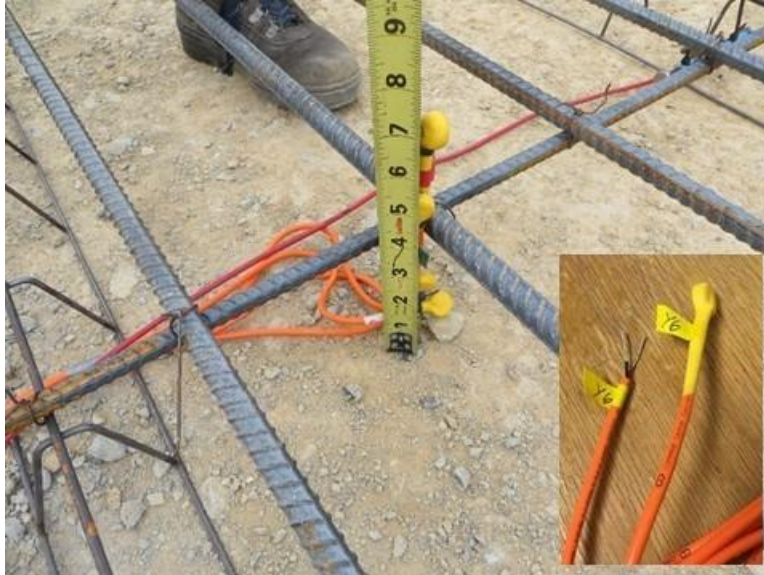
Figure 2. Temperature Measurement Sensors Installation in CRCP. CRCP = continuously reinforced concrete pavement.
