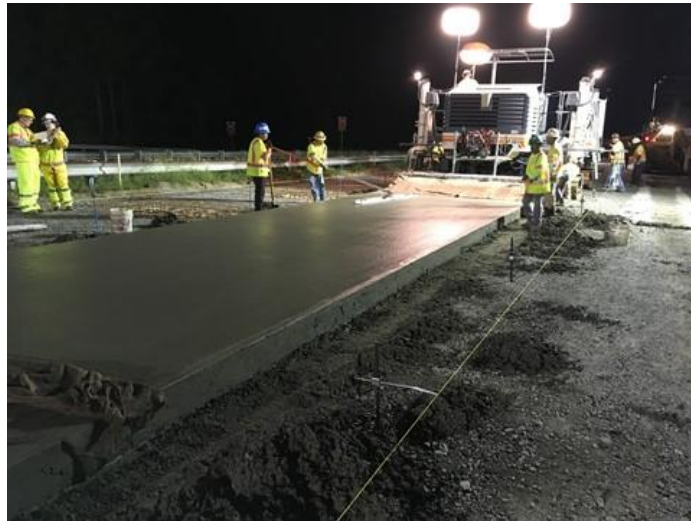
Figure 10. Burlap Drag for Surface Texturing
