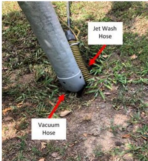
**Figure 4. Clean-out of the Driveway Pipe Shown in Figure 3. Here the jet wash hose is used to loosen and flush out material although the vacuum hose collects it.**
