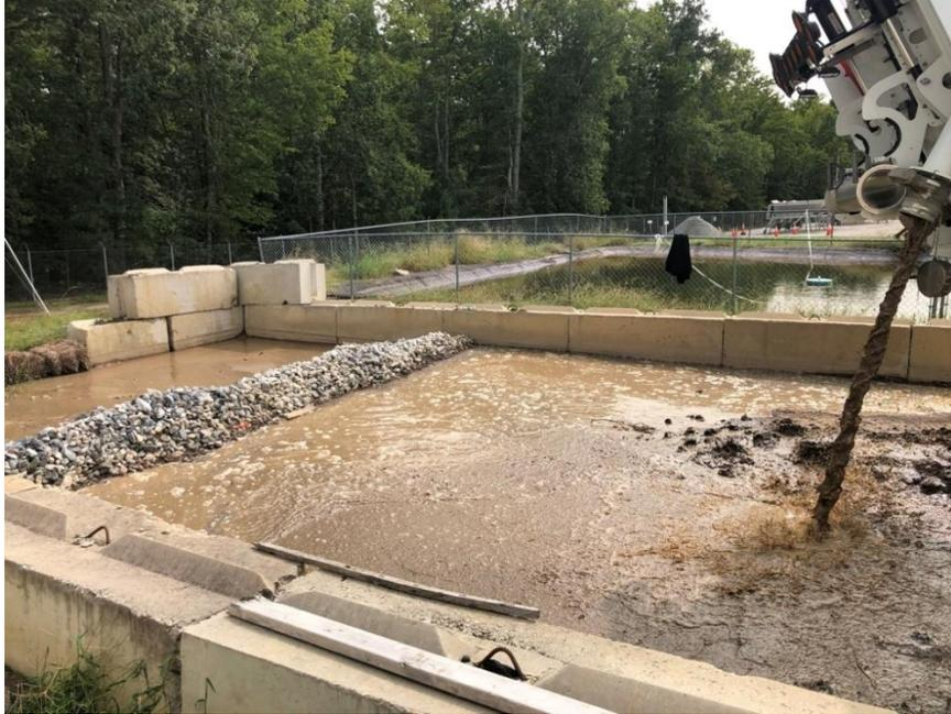
**Figure 5. A Typical Dewatering Pad Used to Drain Material Collected During Storm Drain and Pipe Clean-Outs**
