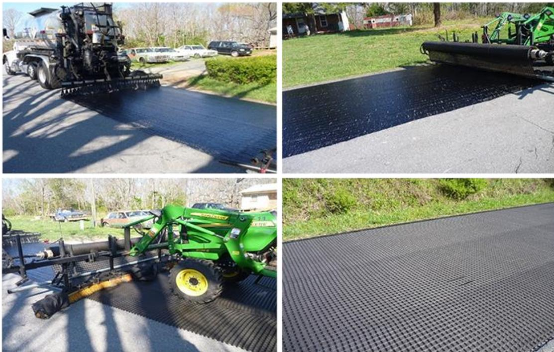
**Figure 2. Interlayer Placement on Route 611**
