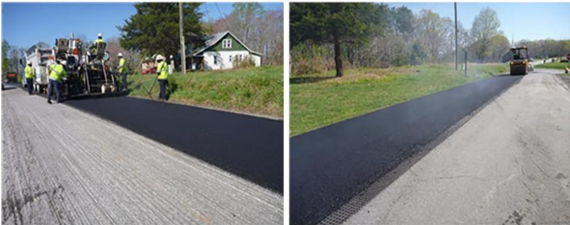
**Figure 4. Asphalt Overlay Placement**
