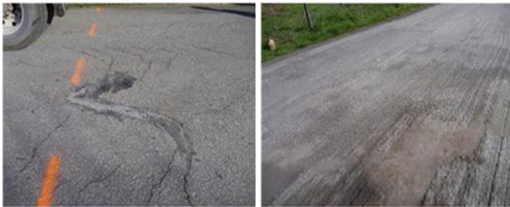
**Figure 1. Slippage Cracks and Milled Surface on Route 611**
