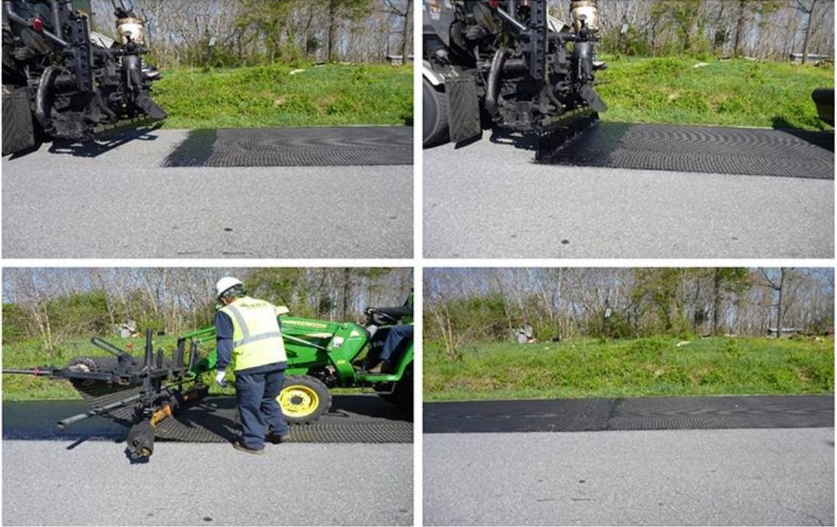
**Figure 3. Longitudinal Interlayer Overlap (Route 611)**
