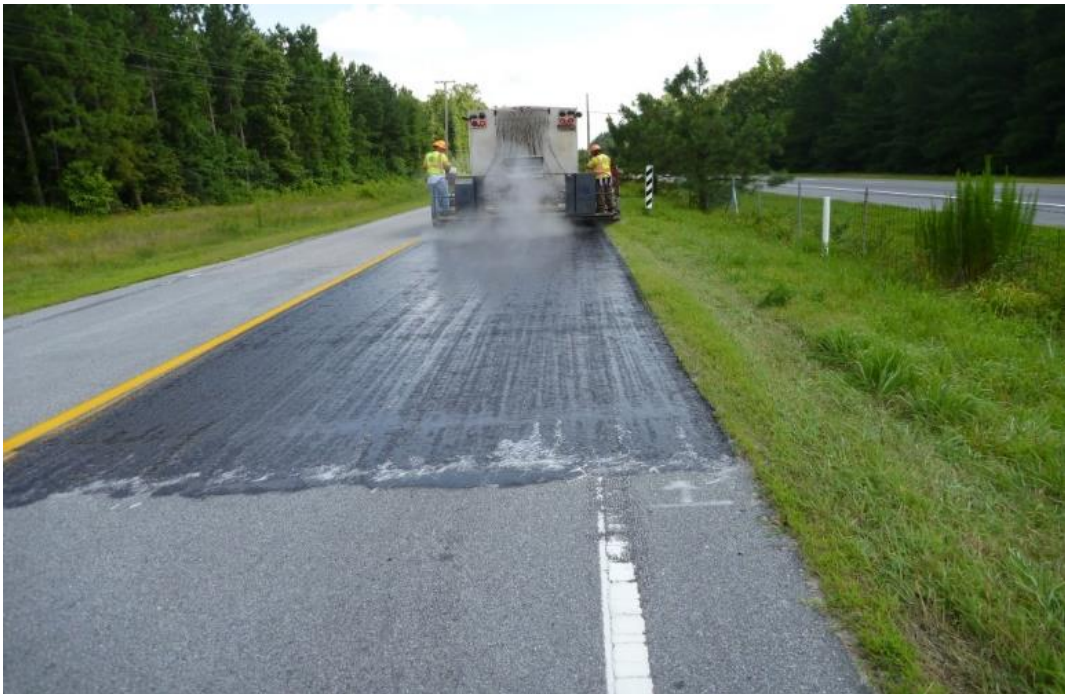
Figure 2. Placement of Fibers and Emulsion
