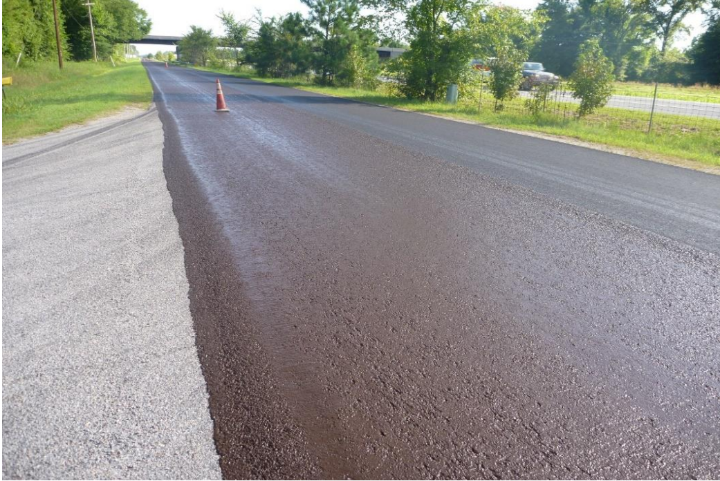
Figure 8. Microsurfacing Before Opening to Traffic
