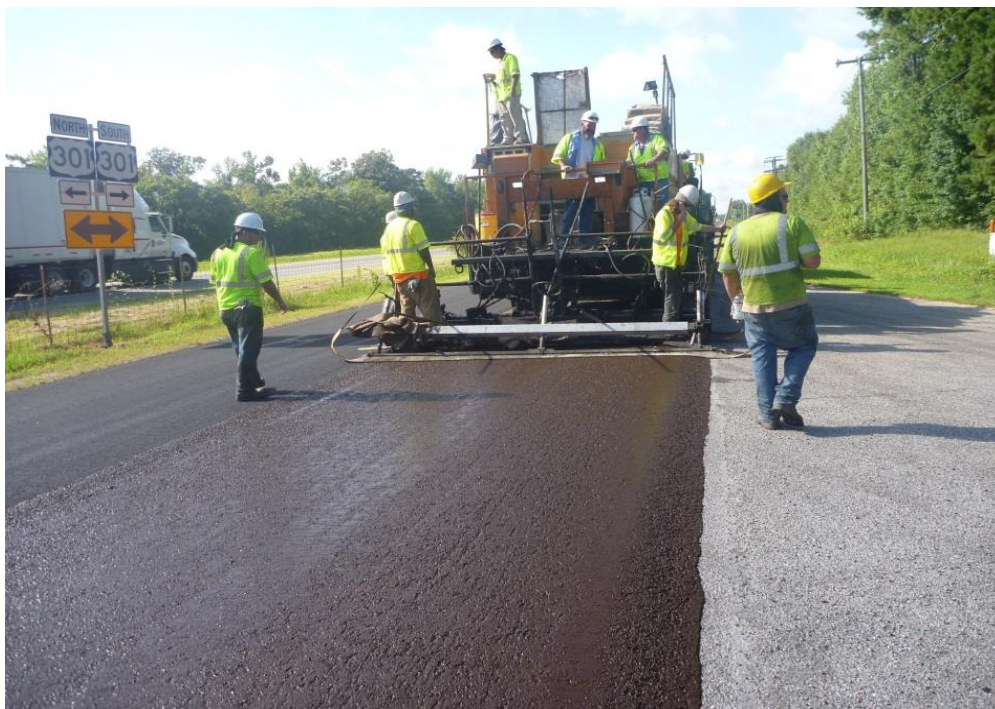
Figure 7. Microsurfacing Placement
