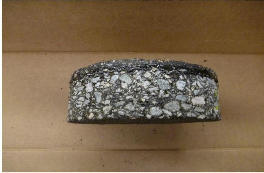
Figure 15. Core Showing FiberMat + Microsurfacing Surface Above Existing Asphalt Top Surface
