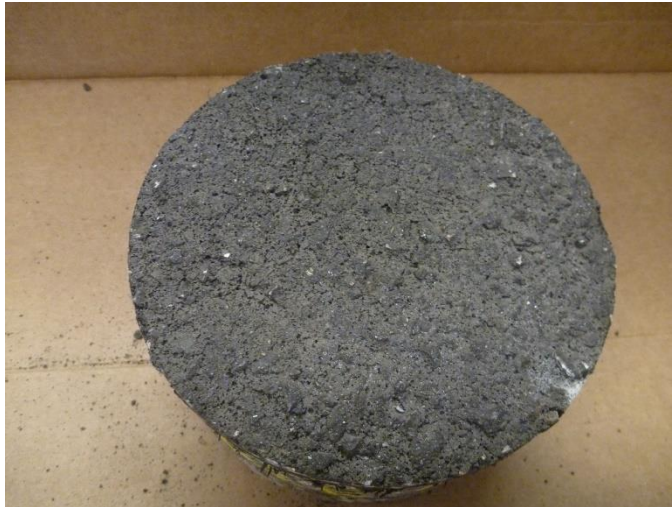
Figure 18. Final Pavement Surface With Microsurfacing
