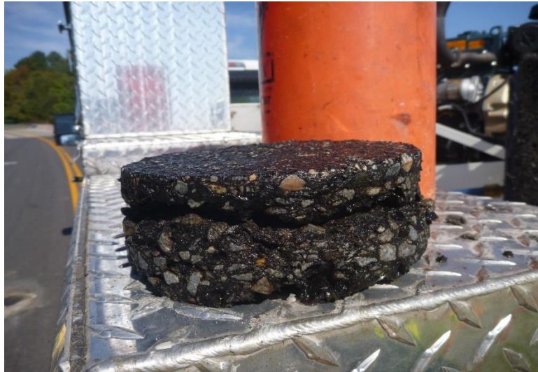
Figure 24. Core Showing Moisture Damage and Delamination
