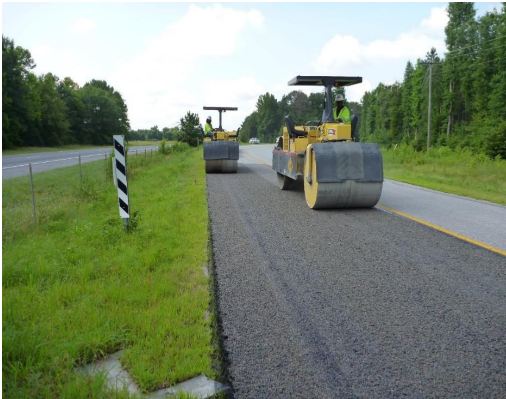
Figure 6. Compaction Using Steel Rollers
