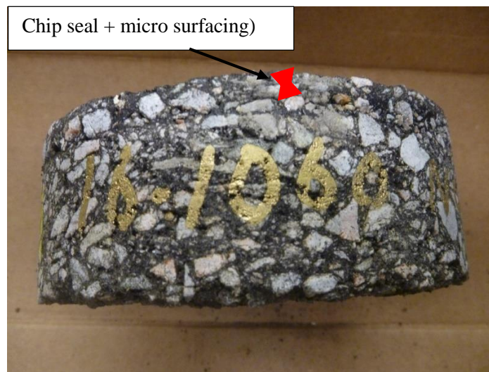
Figure 16. Core Showing Chip Seal + Microsurfacing Above Existing Asphalt Top Surface
