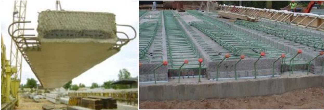
Figure 1. Development of the Inverted T-Beam System, Original Poutre-Dalle System left (reprinted with permission from Matiere, from their website at https://www.matiere-tp.com/beam-slab ), MnDOT System right (Hagen et al., 2005, reprinted with permission)
