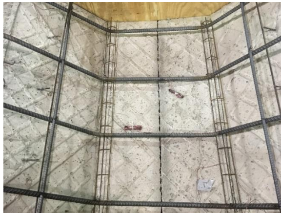
Figure 20. Cross-hatched Surface Roughness with Plastic Sheet as Bond Breaker
