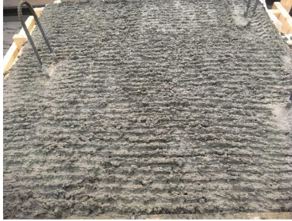
Figure 19. Raked Surface Finish above Extended Web Region
