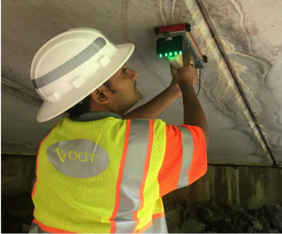
**Figure 28. MFLIS Device Scanning Underside of Box Beam. MFLIS = magnetic flux leakage inspection system.**
