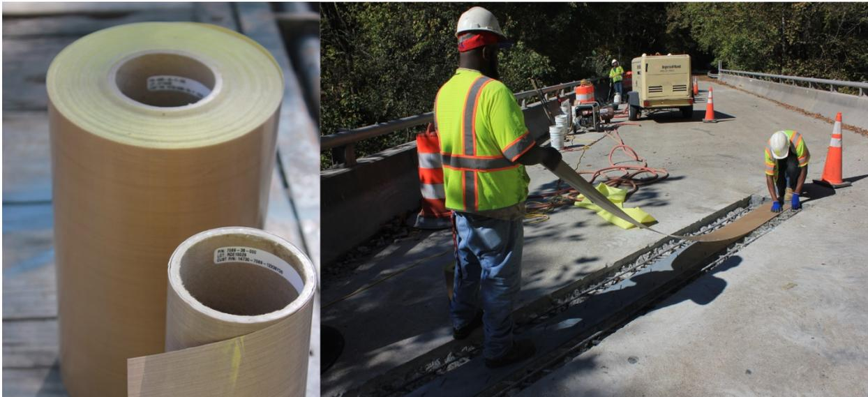
**Figure 12. Debonding Material: *Left*: PTFE-Coated Fabric Roll; *Right*: Installation of Debonding Layer. PTFE = polytetrafluoroethylene.**
