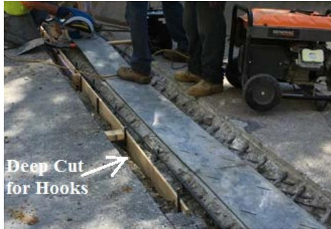
Figure 19. Formation of Elastomeric Concrete Hook
