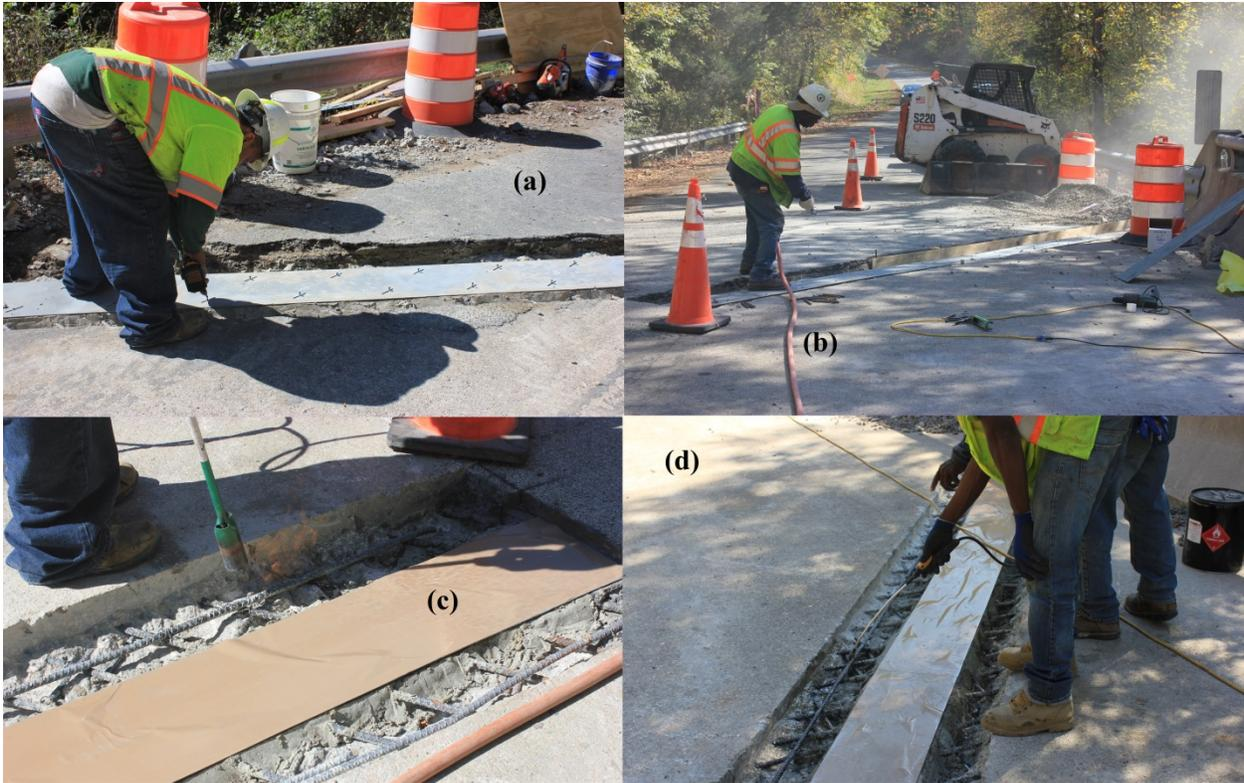
**Figure 11. ECPJ Installation Sequence: (a) Bolting Steel Plate; (b) Cleaning With Compressed Air; (c) Placing Debonding Layer and Heating to Remove Moisture; and (d) Applying Primer. ECPJ = elastomeric concrete plug joint.**
