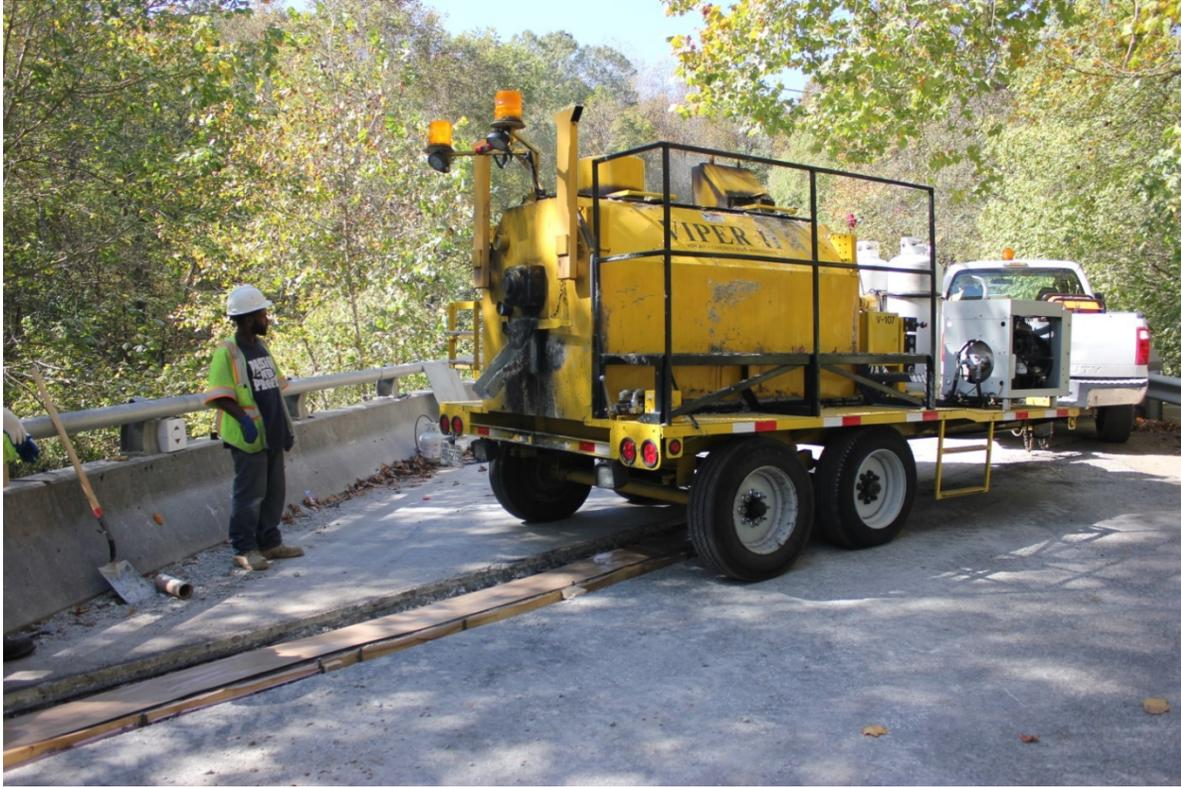
**Figure 13. Preparing to Pour Hot-Applied Elastomeric Concrete**
