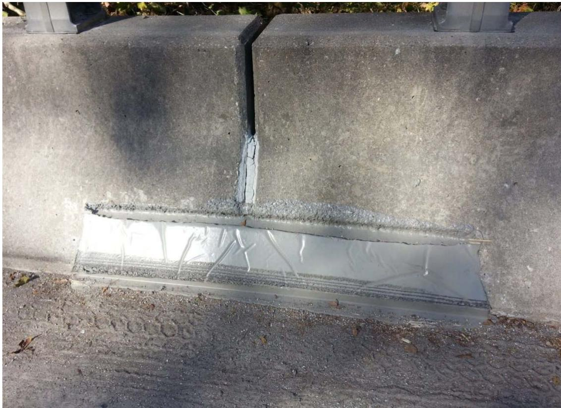
**Figure 14. ECPJ Formed on Parapet Stem. ECPJ = elastomeric concrete plug joint.**
