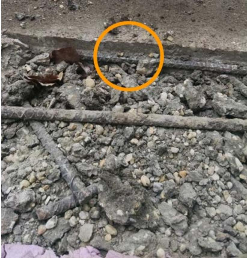
**Figure 21. Low Concrete Cover Over Pier Reinforcing Bar**
