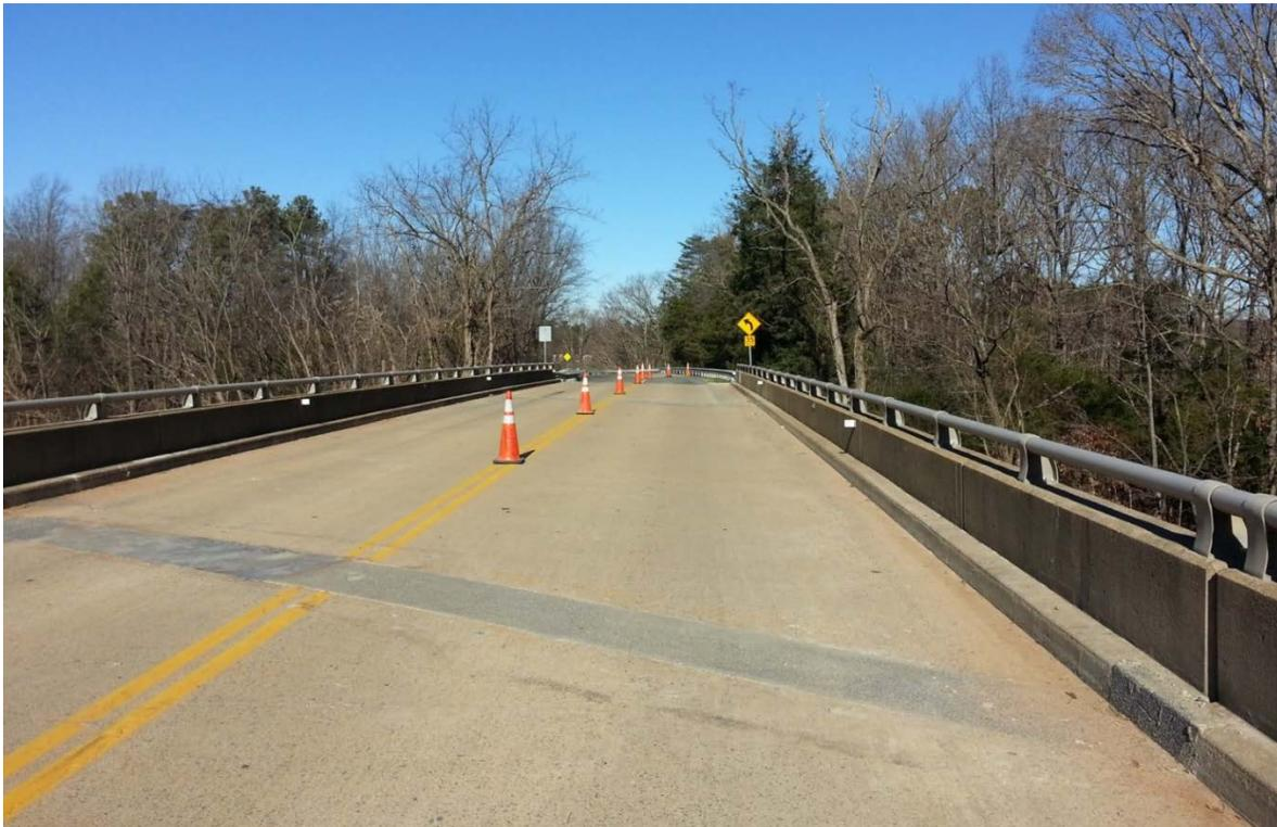
**Figure 16. Bridge Deck With ECPJ System. ECPJ = elastomeric concrete plug joint.**
