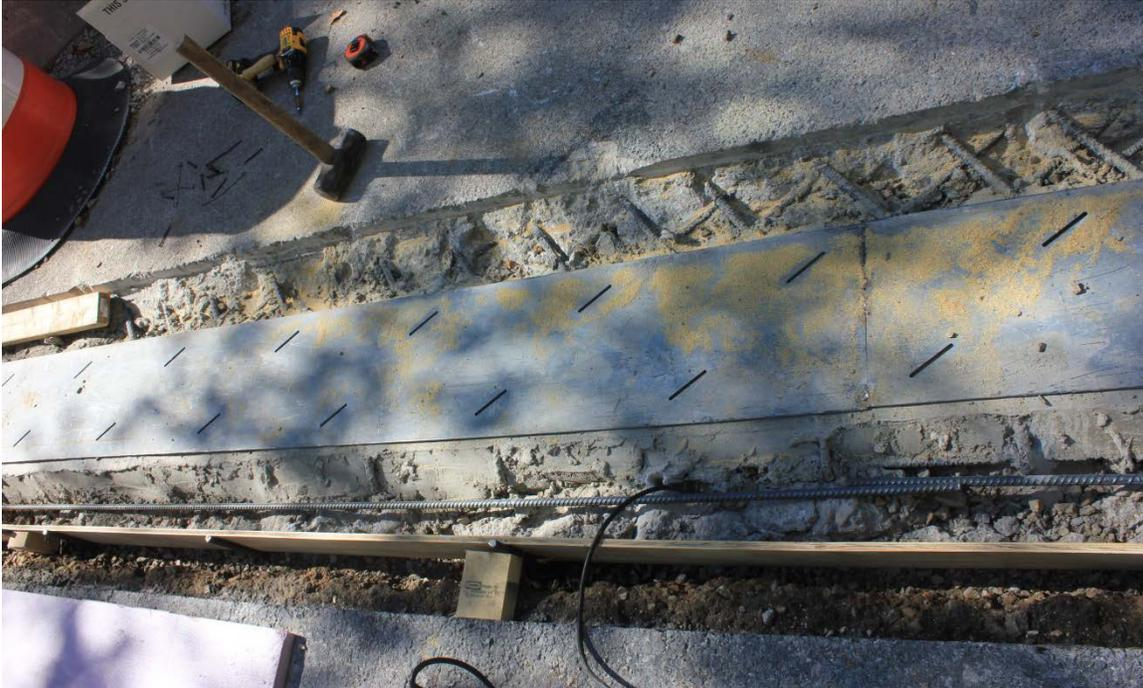
**Figure 10. Preparation of Joint**
