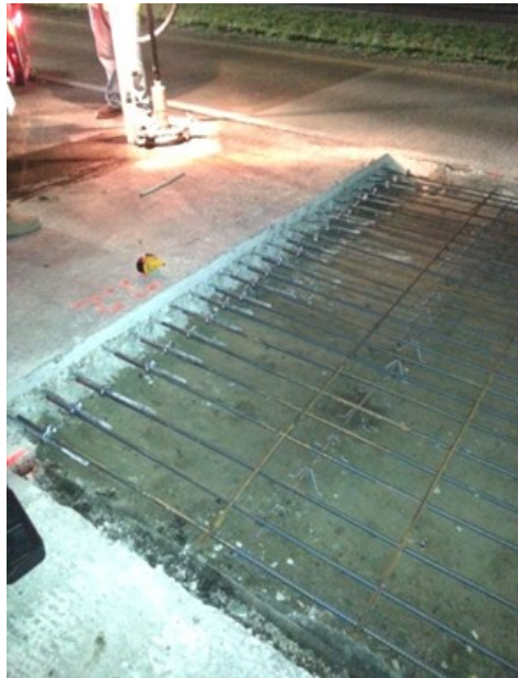
Figure 24. Additional Supports Keeping Steel at Constant Depth on SR 288
