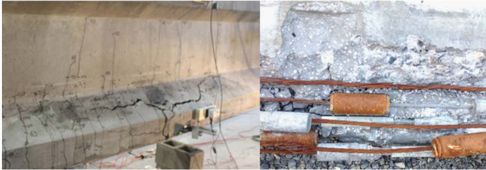
Figure 53. Flexural Cracks in Patch Concrete at Failure (left) and Failed Splices and Strands (right)
