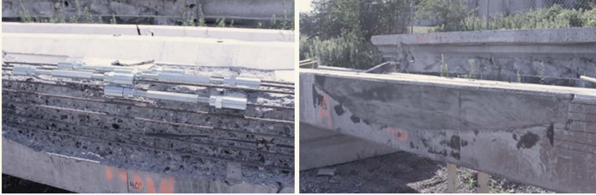
Figure 21. Completed Installation of the Strand Splices and Beam after Form Removal
