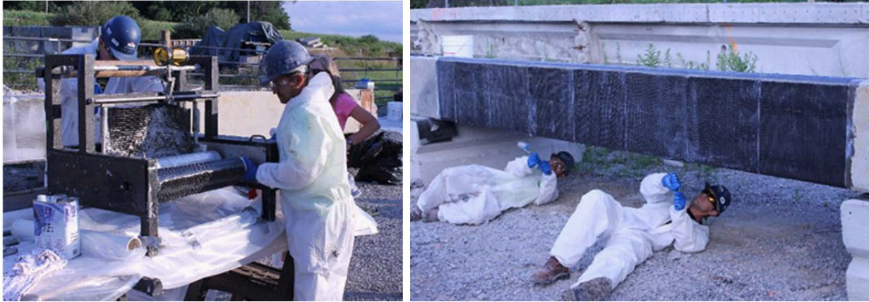
Figure 23. FRP Saturation Process and Rolling of FRP Fabric to Ensure Bond to Concrete
