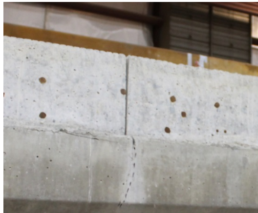
Figure 39. Saw-Cut Gaps in the Deck Concrete of Beam D
