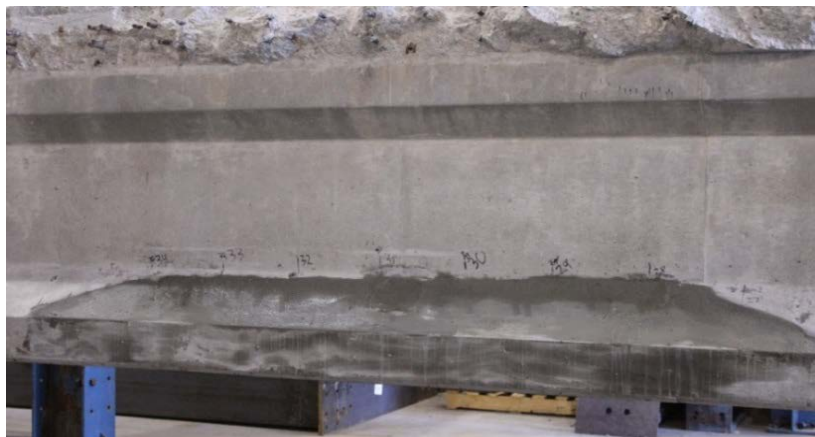
Figure 17. Completed Repair After Form Removal
