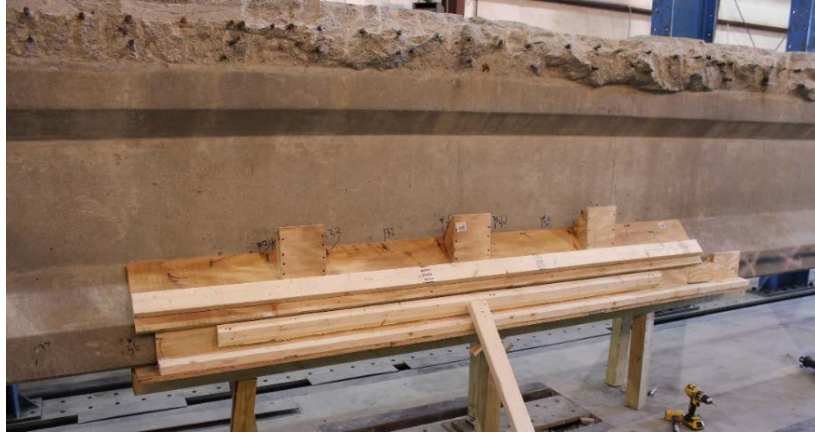
Figure 16. Formwork for Concrete Placement
