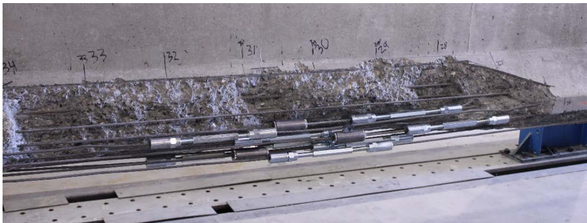
Figure 15. Completed Installation of Strand Splices
