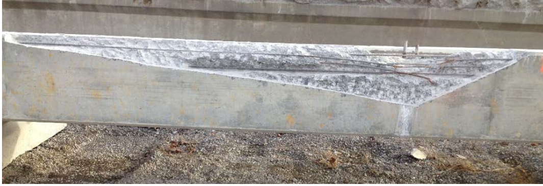
Figure 25. Beam D After Chipping and Saw Cutting
