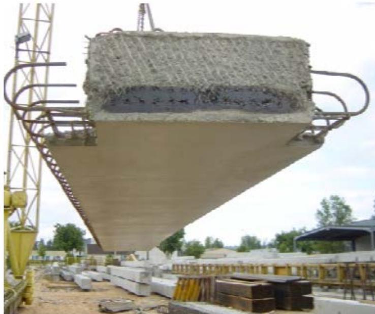
**Figure 1. Poutre-Dalle System. Reprinted with permission from Matiere. From their website at <https://www.matiere-tp.com/beam-slab>.**
