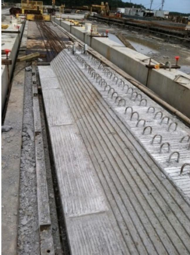
**Figure 28. Roughened Precast Surfaces**
