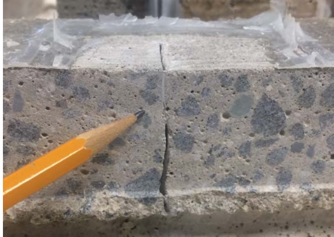
Figure 15. Epoxy Restricting the Opening to the Rebar in an Unsealed Specimen
