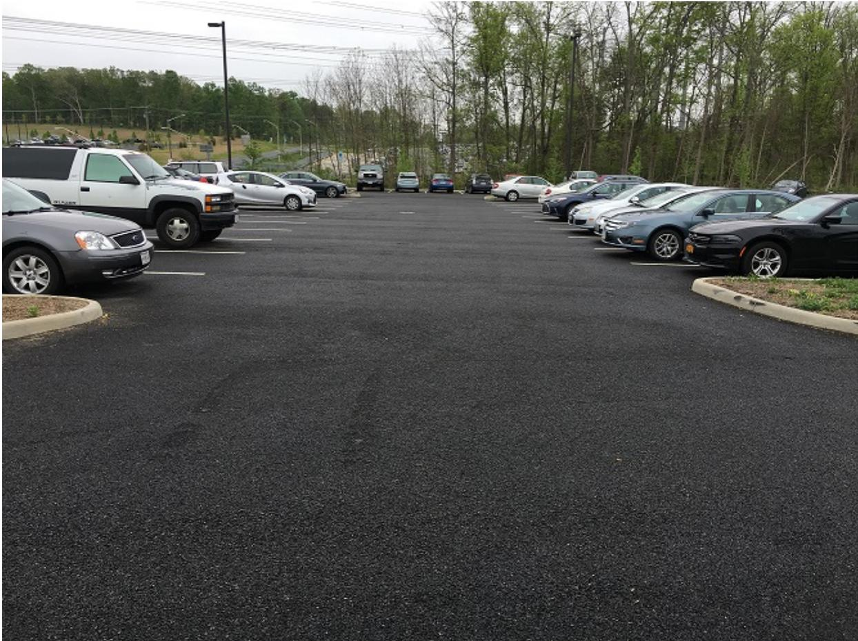
**Figure 1. Completed Porous Asphalt Park & Ride Facility**
