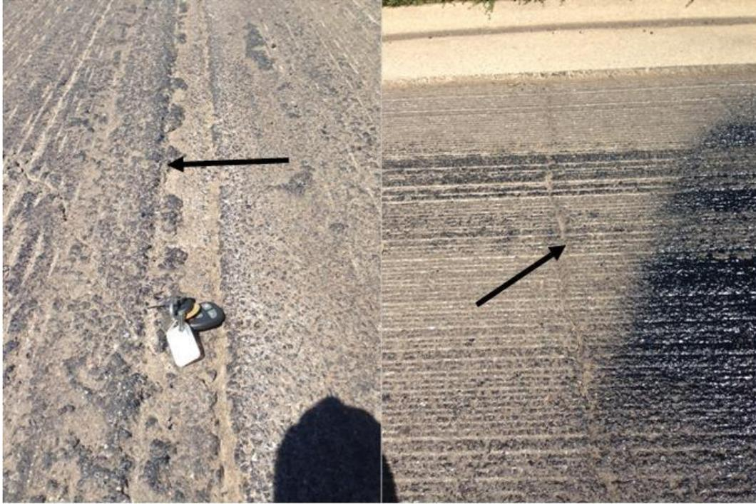
**Figure 3. Milled Surfaces (*left and right*) and Typical Cracking (*right*). The image on the *left* shows the joint between passes of the paver from the original paving project, and the image on the *right* shows a typical transverse crack.**
