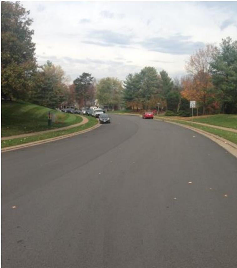
**Figure 15. Photograph Taken of Summerwood Circle on November 6, 2015, 15 Months After Completion of the Project. To the *left* of the longitudinal joint is the control section; to the *right* is the HP (high polymer) section.**
