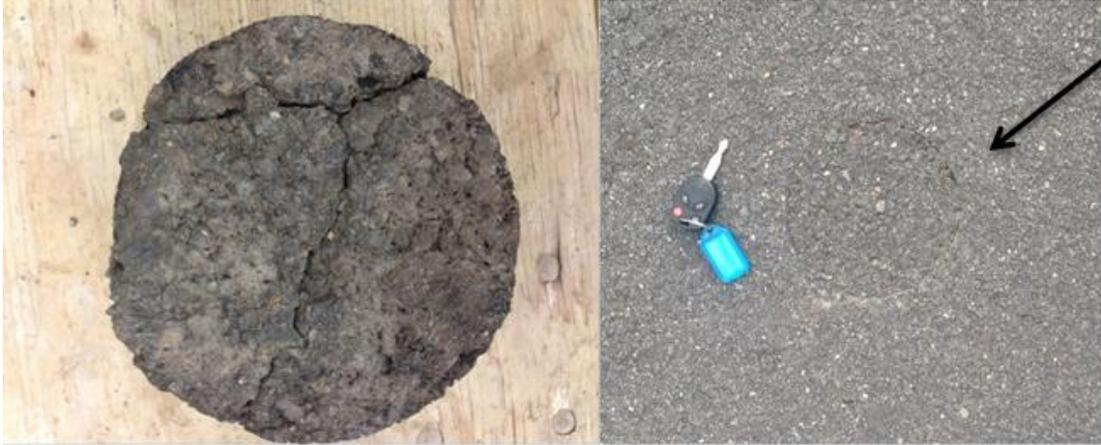
**Figure 16. Bottom of Core Taken at Construction Showing Cracked Underlying Pavement Structure Beneath Experimental Section (*left*) and Subsequent Core Hole and Patch After 15 Months in Service (*right*)**
