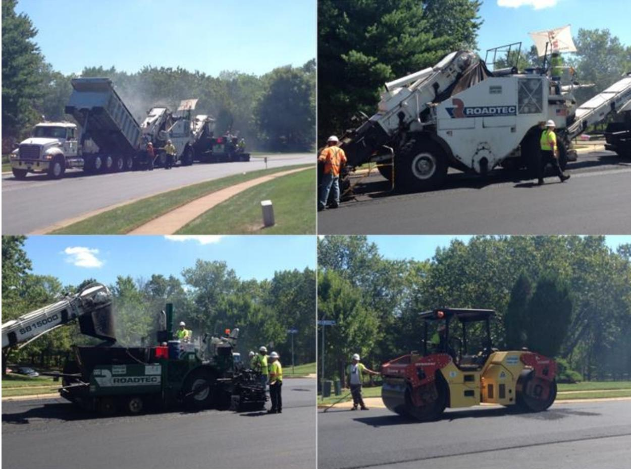
**Figure 5. Each Phase of Paving Operation. *Top left: pavement train; top right: material transport vehicle; bottom left: material transport vehicle feeding paver; bottom right: the roller.***
