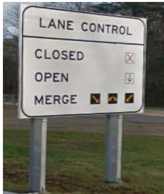
Figure 8. Available Lane Use Control Signals on I-66
