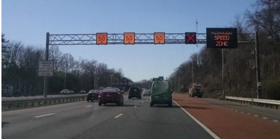
Figure 7. Example of Gantry With ATM Techniques. ATM = Active Traffic Management.
