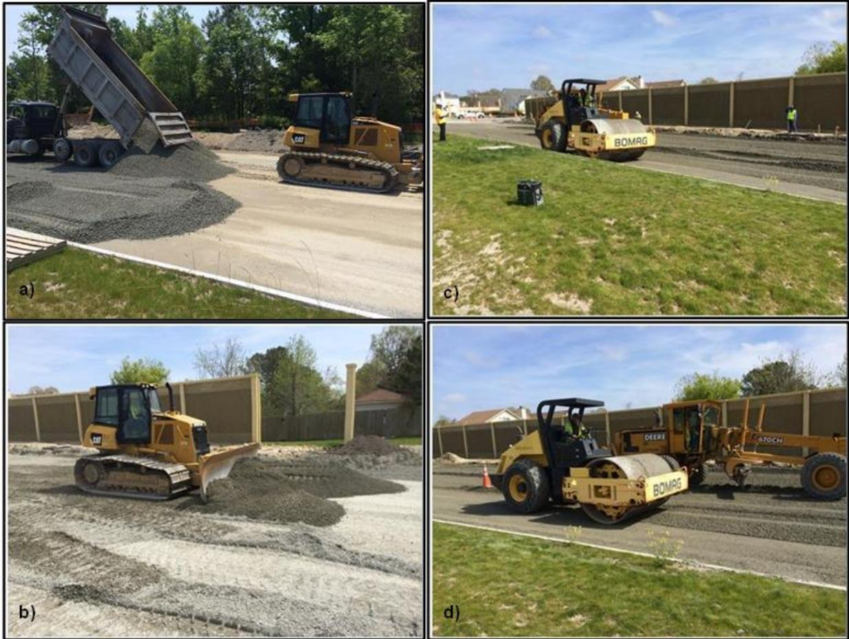
**Figure 5. CTA Construction at Nimmo Parkway: (a) back dumping CTA; (b) spreading CTA with motor grader; (c) compaction with roller; (d) grading to 8-in thickness using blade and re-compacting. CTA = cement-treated aggregate.**
