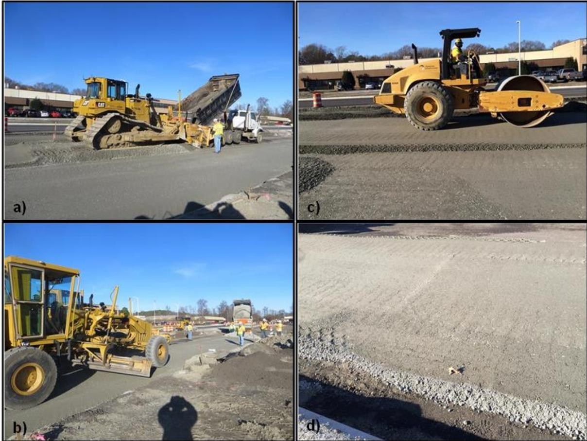
Figure 3. Construction of CTA on Middle Ground Boulevard: (a) haul truck dumping to spreader; (b) blading with motor grader and back dump; (c) compaction with vibratory roller; (d) finished CTA surface. CTA = cement-treated aggregate.
