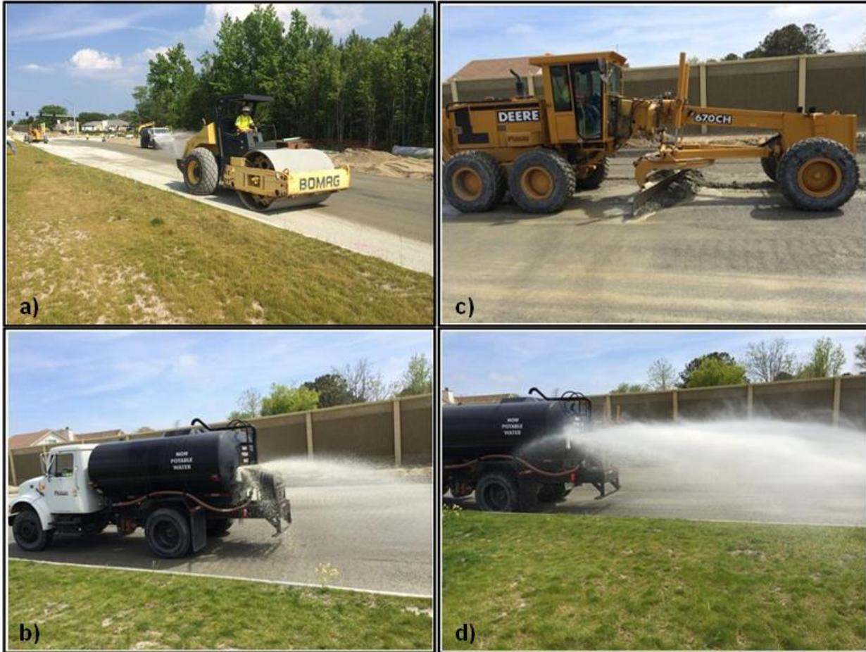
Figure 6. Water Spray, Grading, and Re-compaction of CTA on Nimmo Parkway: (a) dry CTA surface; (b) water truck to wet surface for more compaction; (c) blading to achieve proper grade and standing water; (d) heavy water spray. CTA = cement-treated aggregate.
