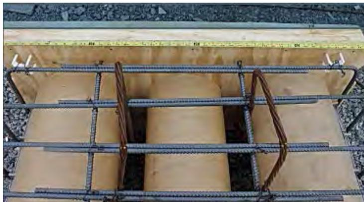
Figure 10. Voided Slab Formwork and Reinforcement Cage
