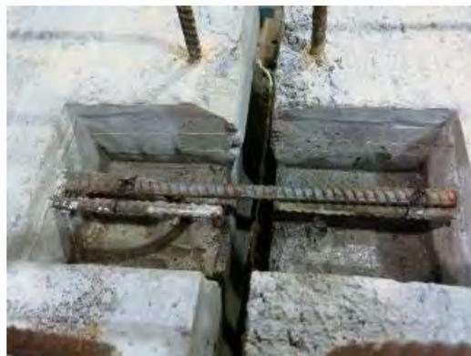
**Figure 15. Blockout With Tied in Lap Splice Bar Before UHPC Placement**
