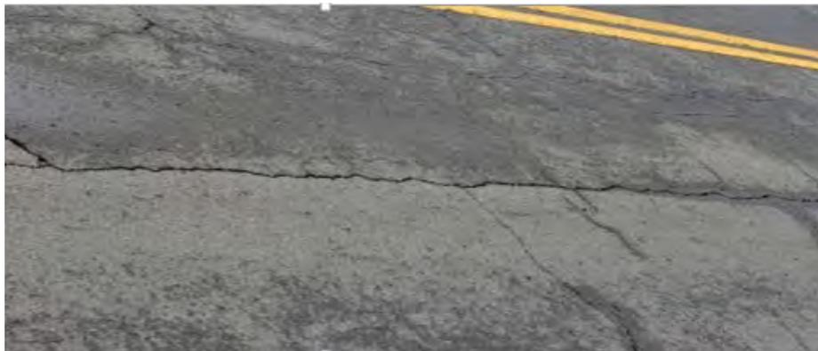
**Figure 3. Longitudinal Reflective Cracking in Asphalt Overlay**
