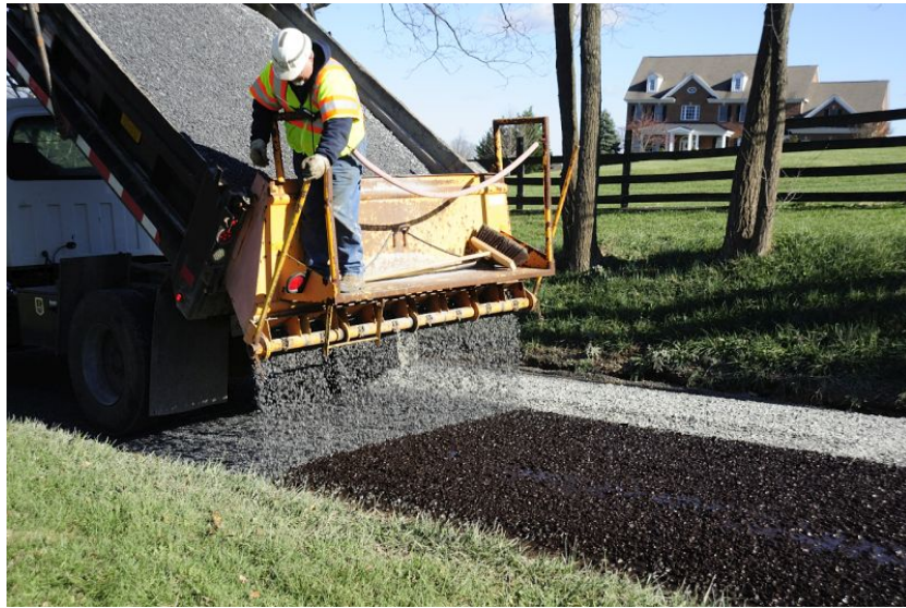
Figure 7. Chip Seal Application on Hurley Lane
