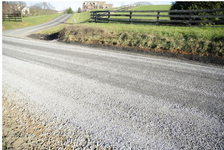
Figure 8. Final Road Surface on Hurley Lane
