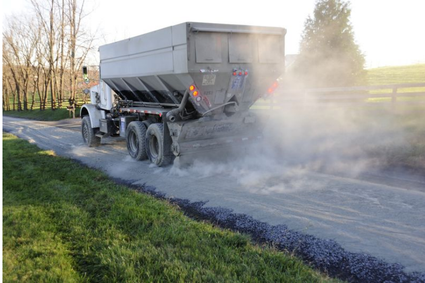
Figure 2. Spreading Cement Stabilizer
