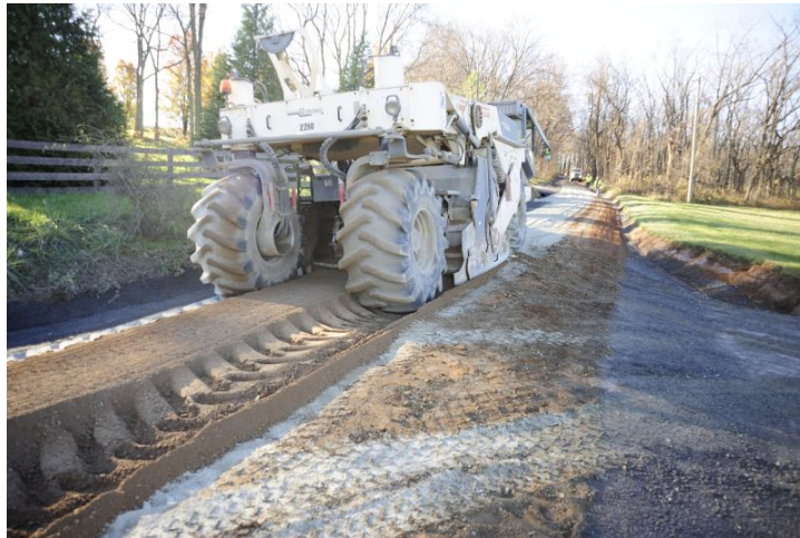
Figure 3. Blending Cement With Wirtgen Reclaimer
