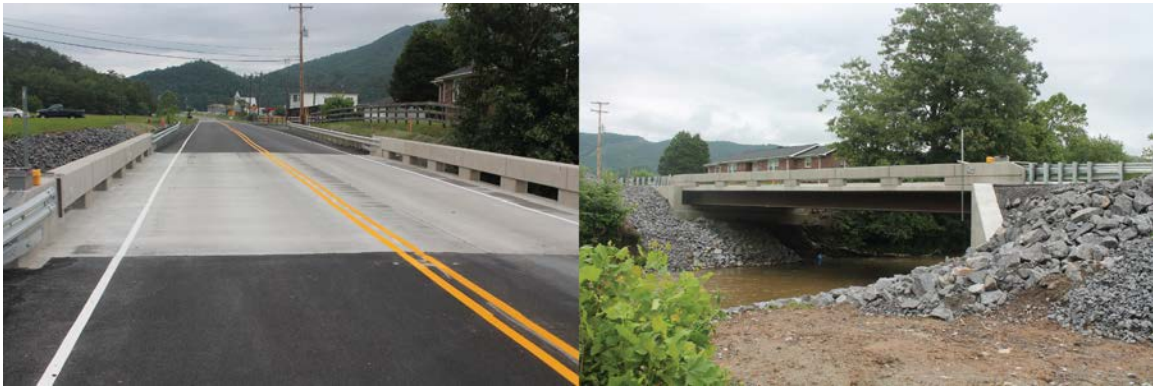
Figure 1. US52 Bridge Deck Constructed With ASTM A1035 CS Steel Bars
