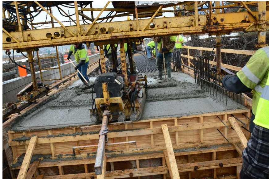
Figure 3. Concrete Placement for Phase I Construction
