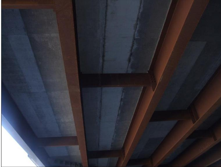
**Figure 30. Underside of I-95 Bridge Over Hermitage Road Showing Beams, Diaphragms, and Joints After Superstructure Replacement Was Completed**
