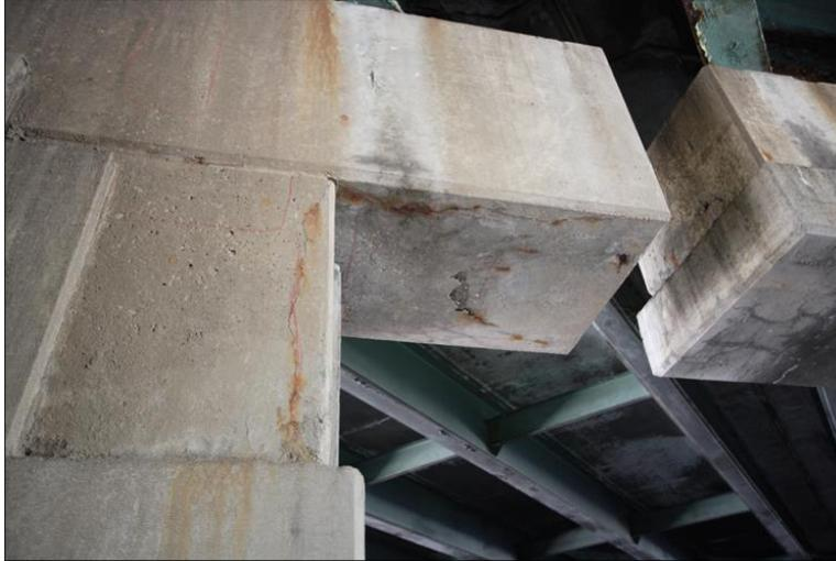
**Figure 34. Rust Stains From Water Dripping Onto Caps and Corrosion Damage on Underside of Cap Supporting I-95 Bridge Over Hermitage Road Before Repair. Tight cracks can also be seen on the underside of the cap on the right. Photograph courtesy of VDOT Public Affairs.**
