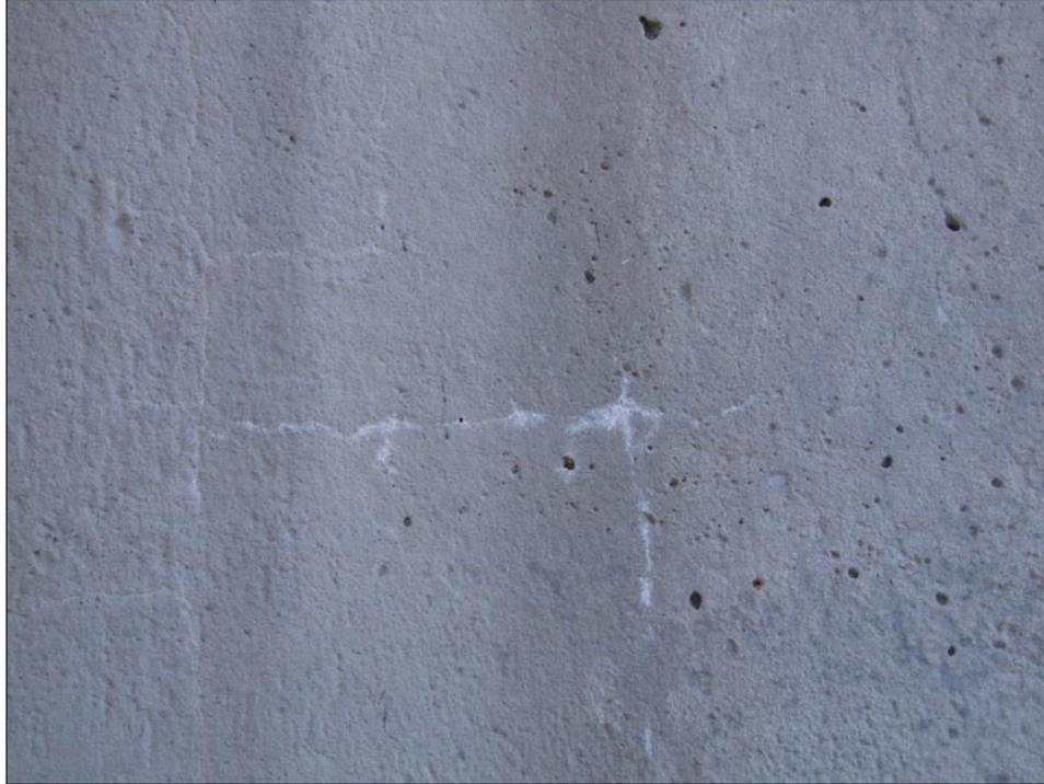
**Figure 37. Previously Existing Crack in Concrete Exhibits Mineral Deposit, Possibly Forming During ECE Treatment of I-95 Bridge Over Hermitage Road. ECE = electrochemical chloride extraction.**
