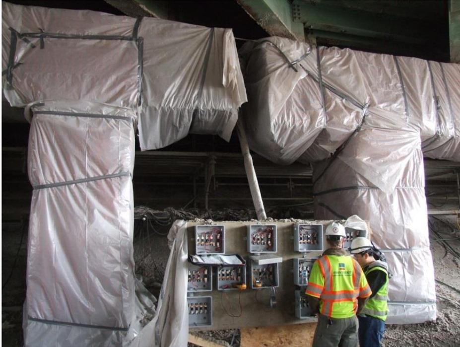
**Figure 21. ECE on I-95 Bridge Piers.** To ensure better control and an even current distribution during ECE treatment, the electrical systems are divided into smaller areas (sub-zones) on each substructure element. These sub-zones are being monitored during treatment and electric measurements recorded by a qualified technician. ECE = electrochemical chloride extraction.
