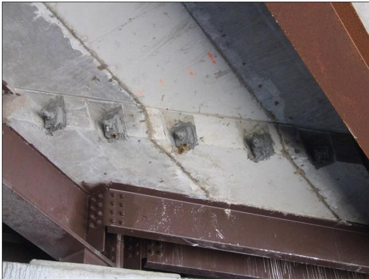
**Figure 31. Underside of I-95 Bridge Over Hermitage Road Showing Post-Tensioning Termination Points After Superstructure Replacement Was Completed. No leaking joints were observed.**
