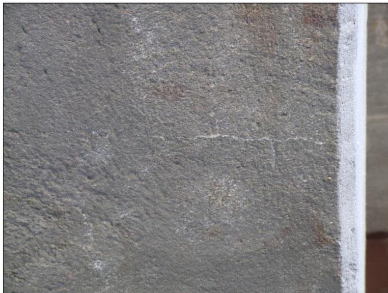
**Figure 44. I-95 Bridge Over Overbrook Road Showing Mineral Deposit on Column After ECE. ECE = electrochemical chloride extraction.**
