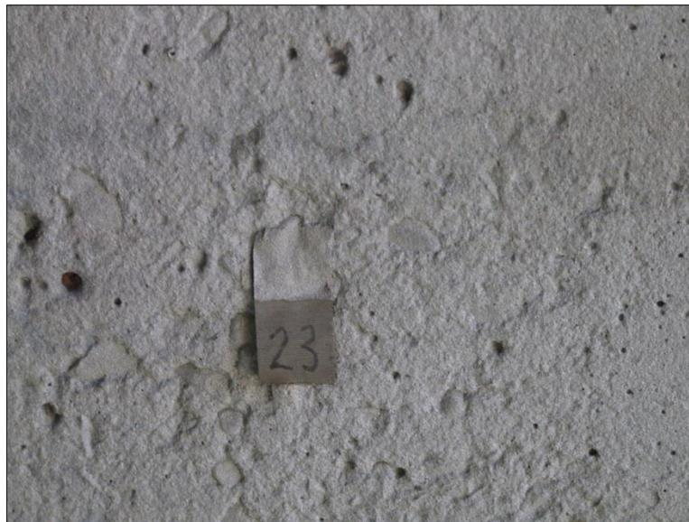
**Figure 36. I-95 Bridge Over Hermitage Road Concrete Surface Substructure Element After Application of Al-Zn-In Coating for GACP. GACP = galvanic anode cathodic protection.**
