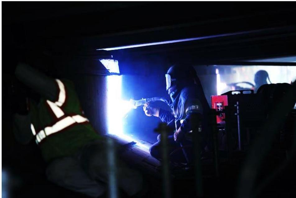
**Figure 28. Photograph Taken in December 2011 Showing Arc Spraying of I-95 Bridge Abutment Along Hermitage Road. Molten Al-Zn-In is being applied to the surface of a reinforced concrete element by the arc spray process. Photograph courtesy of VDOT Public Affairs.**
