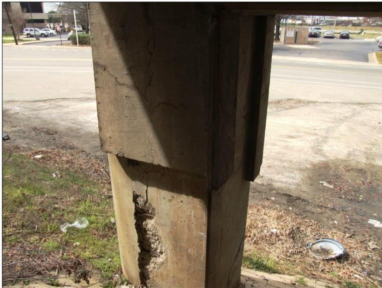
**Figure 33. Corrosion Damage Resulting in Spalling of Column Supporting I-95 Bridge Over Hermitage Road Before Repair**
