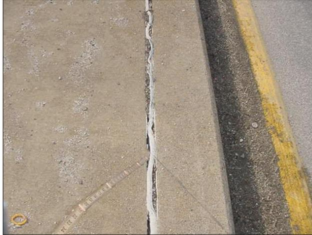
**Figure 7. Photograph From VDOT Inspection Report. The report stated: "Note heavy deterioration of joint seal & spalling along the edges of longitudinal joint in median" (VDOT, unpublished data, 2006).**
