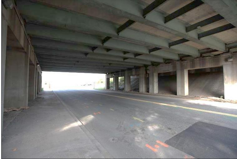
Figure 38. Underside of I-95 Bridge Over Overbrook Road Before Superstructure Replacement and Corrosion Mitigation Work Began. Photograph courtesy of VDOT Public Affairs.
