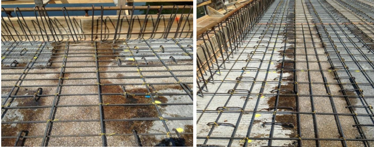
Figure 1. Box Beam Joints With Fiber Strips
