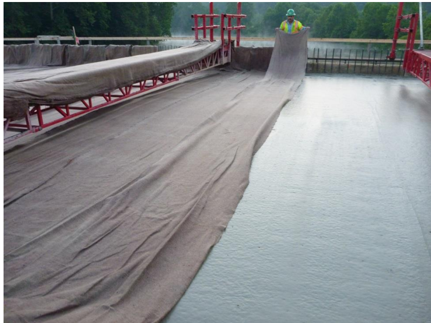
Figure 3. Wet Burlap Placement Immediately After Screeding and Compaction
