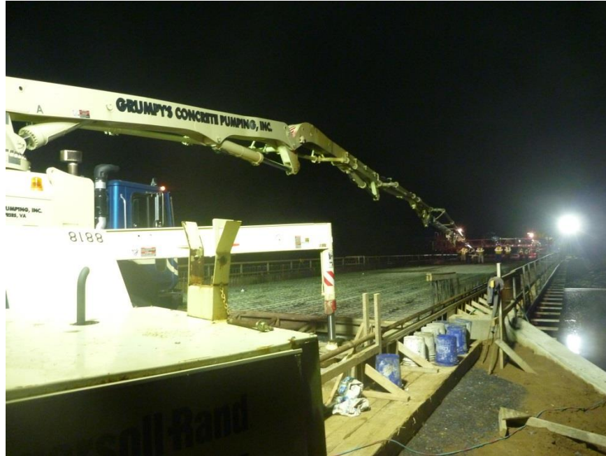
Figure 2. Concrete Placement by Pumping
